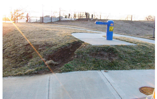
FIGURE 5.32: Erosion is occurring on the south side, as skaters ride directly from the path down the grass.
