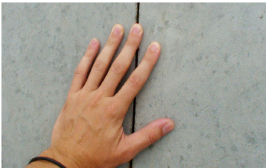
FIGURES 5.60 and 5.61: The correct troweled finish of skate park concrete, and an incorrect sidewalk broom finish.
