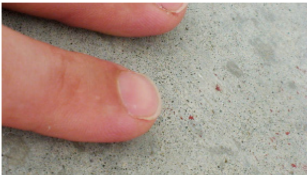
FIGURE 5.34: The surface texture of well-finished concrete is perfect for urethane wheels.
