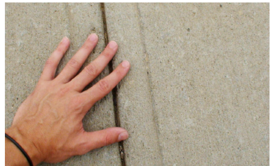
FIGURES 5.60 and 5.61: The correct troweled finish of skate park concrete, and an incorrect sidewalk broom finish.
