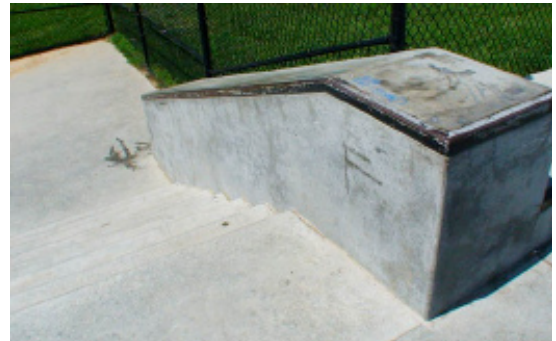
FIGURE 5.53 and 5.54: Square coping should be used on street obstacles.
