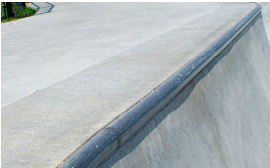
FIGURE 5.55 and 5.56: Round steel coping. Andy Brayman grinding poured concrete pool coping.
