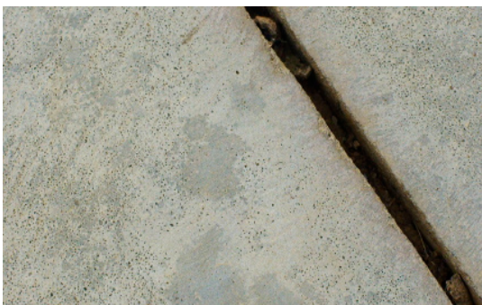
FIGURES 5.62 and 5.63: A correct 1/8” sawn concrete joint, and the author using the surface for controlled
