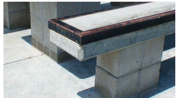
FIGURE 2.20: Square steel coping set into a bench at the Kansas City Skate Plaza.
