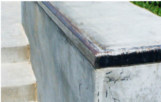
FIGURE 5.53 and 5.54: Square coping should be used on street obstacles.
