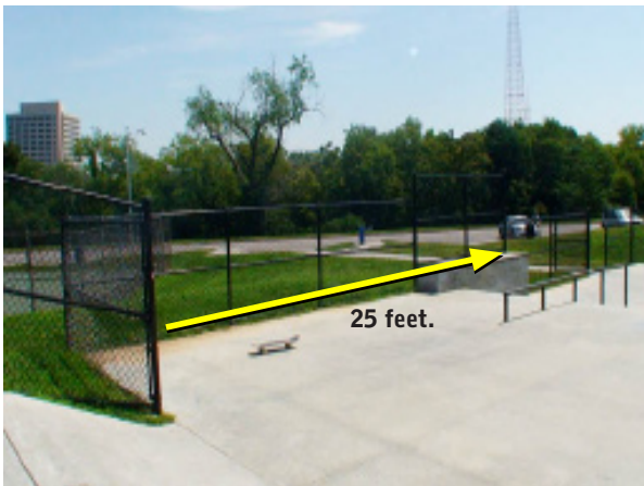
FIGURE 5.38: An example of a run up to a stair set that has too little flat area (about 25'), and the technique of run and drop within the street area.
