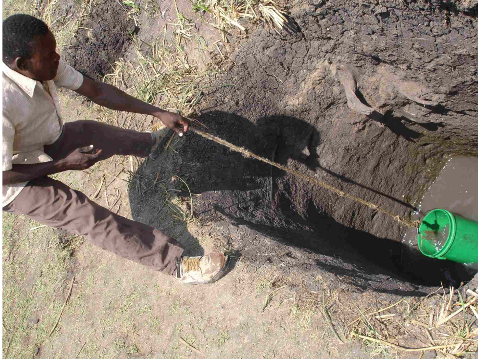
Figure 5. 4: A well dug on the river bed ( longobesi )
