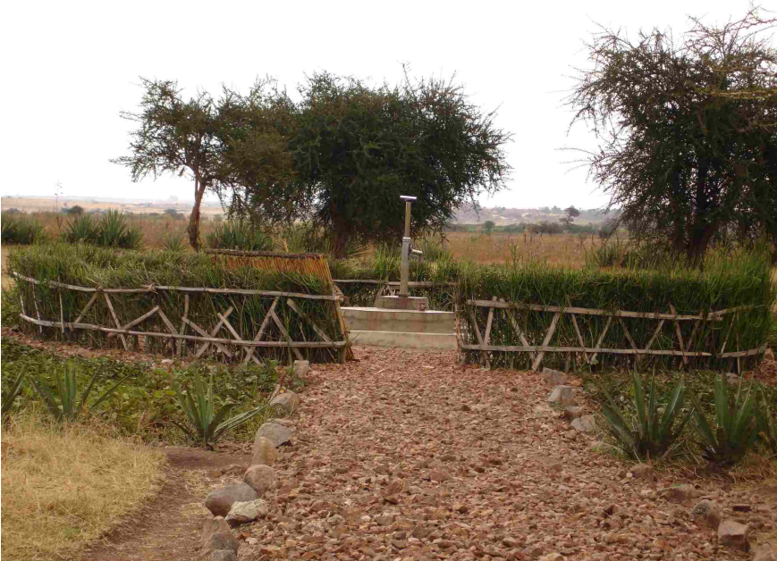
Figure 6. 8: A water pump with a live fence around it
