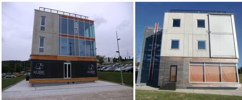
Fig 1 Kubik by tecnalia research facility. General view (left) & specific façade used for the experiment (right)
