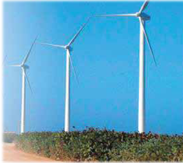
Fig. 1. 9 Three bladed horizontal Axis wind turbine [9].
