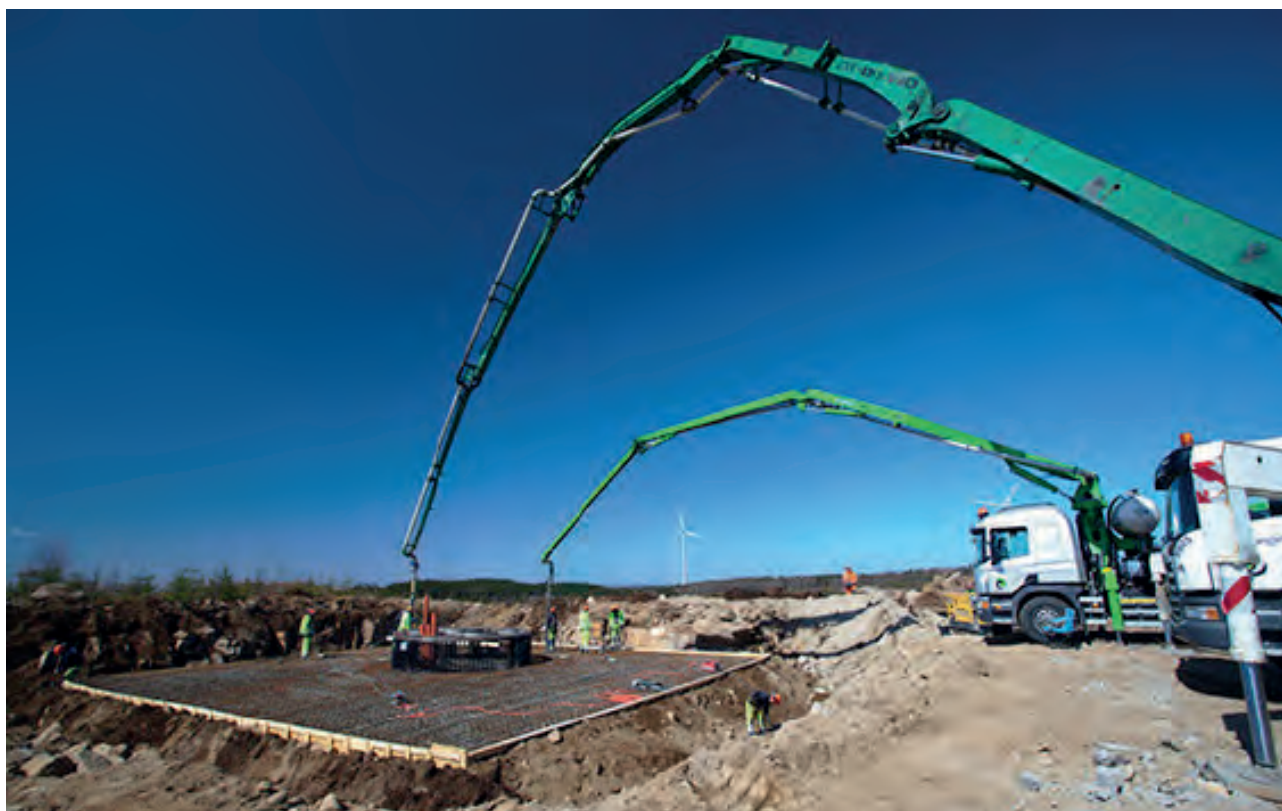
Figure 5: Wind farm construction - pouring concrete for a wind turbine foundation.
