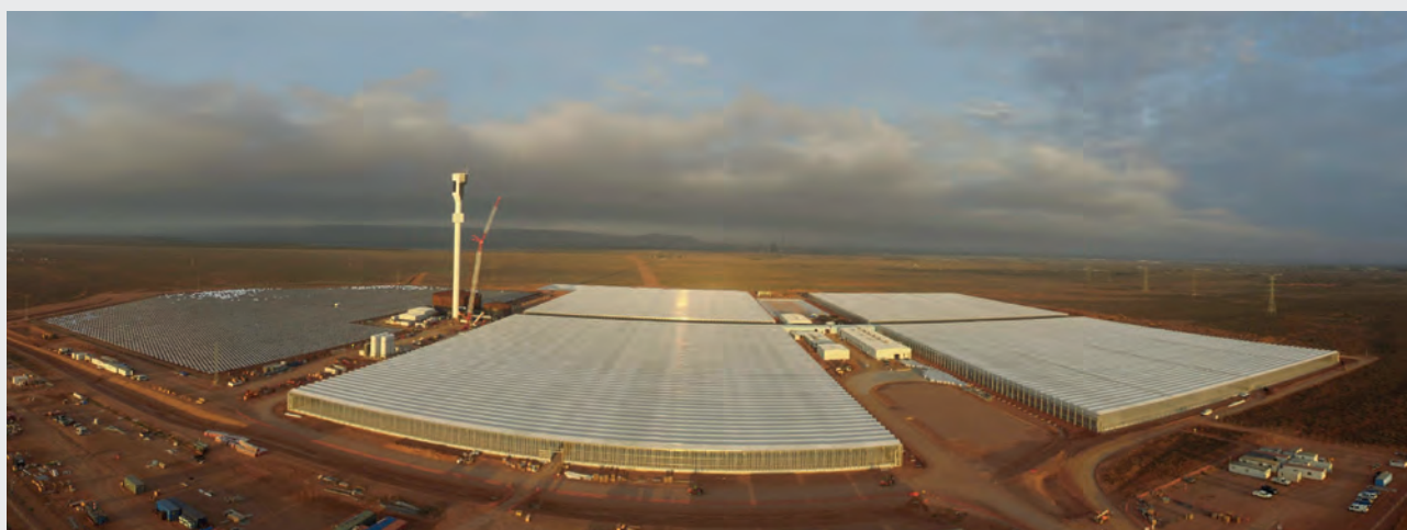
Figure 13: Sundrop Farms Solar Thermal.
