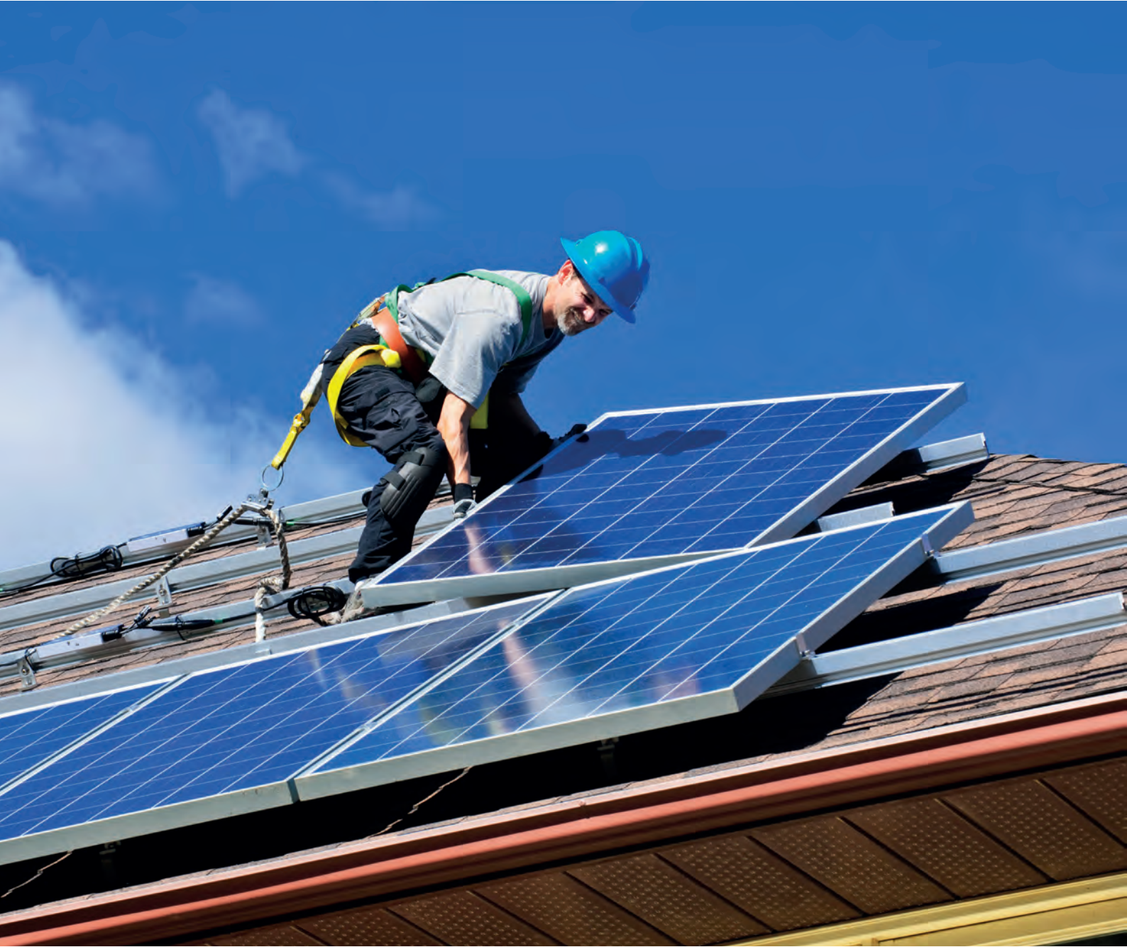
Figure 12: Installing rooftop solar.
