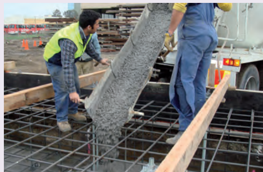
E-Crete uses waste fly ash and slag to achieve a comparable cement for an 80 per cent emissions reduction. Image provided by Zeobond.
