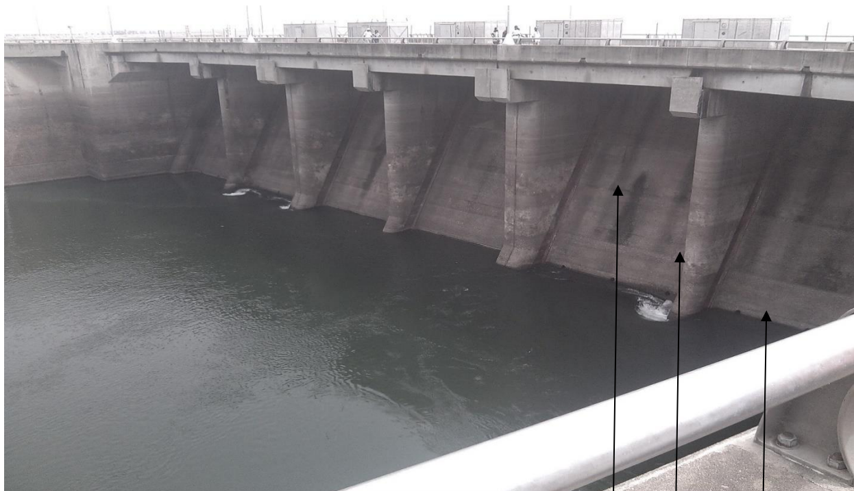
Figure 15: The various levels of water marks on the Akosombo dam during the different seasons. Source: Author, 2021.
