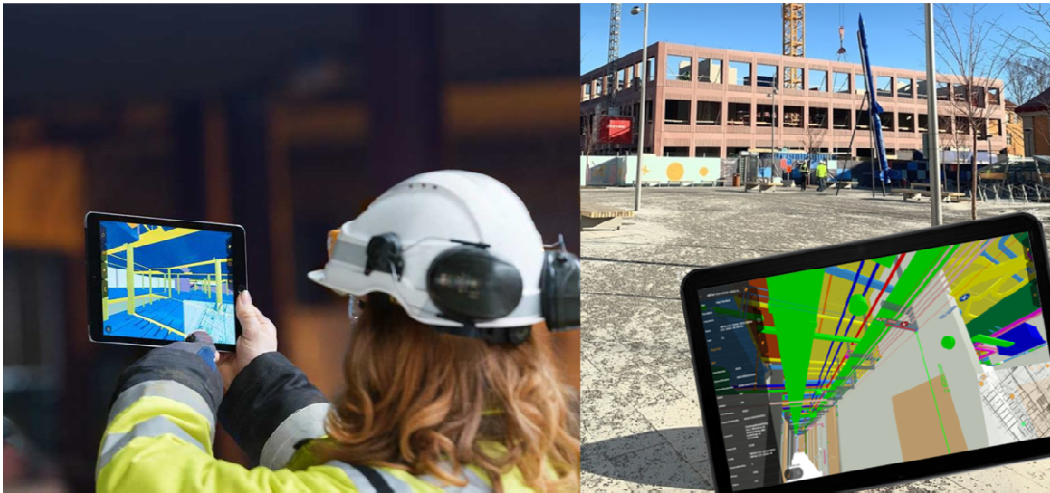
Fig. 3: Left: Use of StreamBIM on-site. Right: View of the Celsius project during construction
