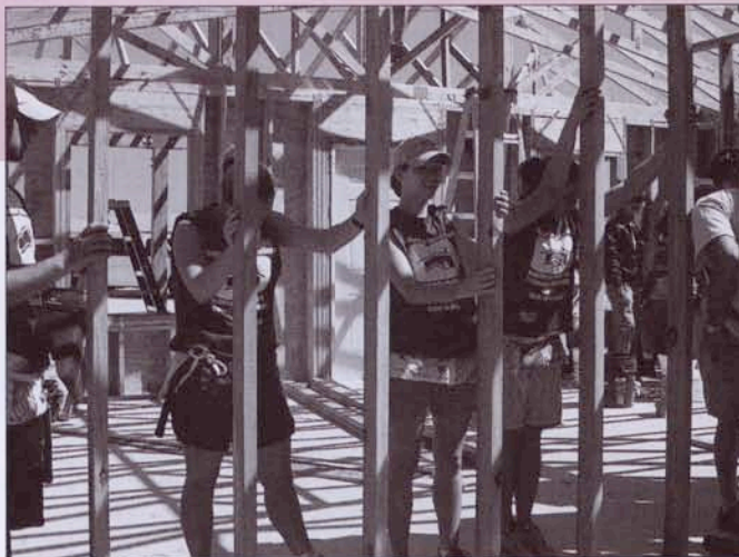
BSC students work on an Habitat for Humanity house in Florida.
