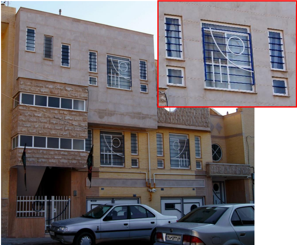
Figure 27. Façade of Mrs. Mz114's house
