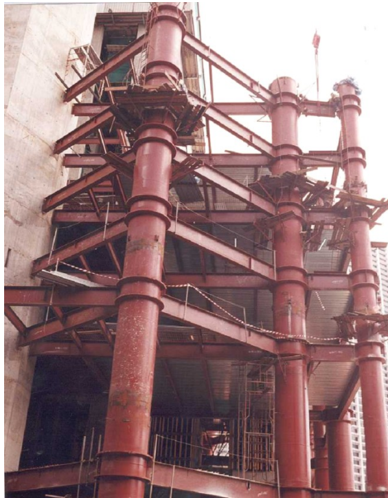
Figure 1.7: Hollow circular steel columns before infilling with concrete (Liew, 2004)
