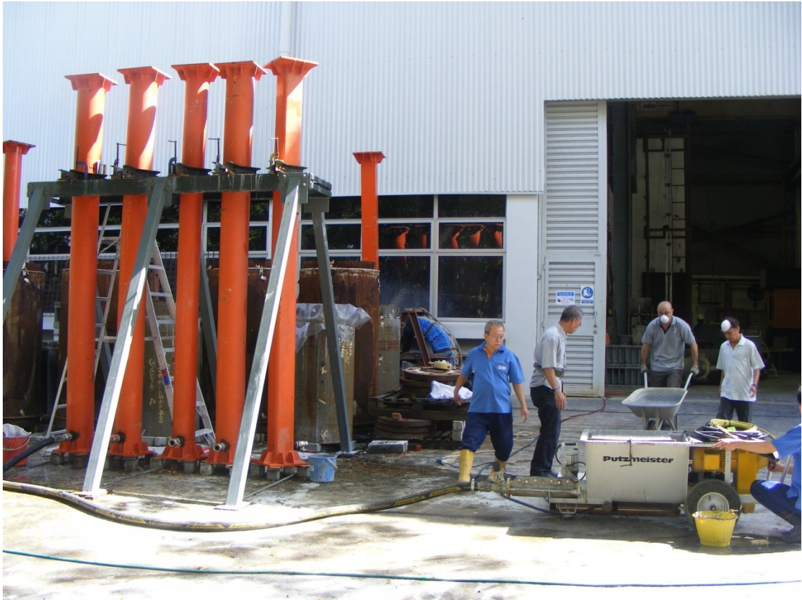
Figure 5.1: Casting of UHSC by pumping
