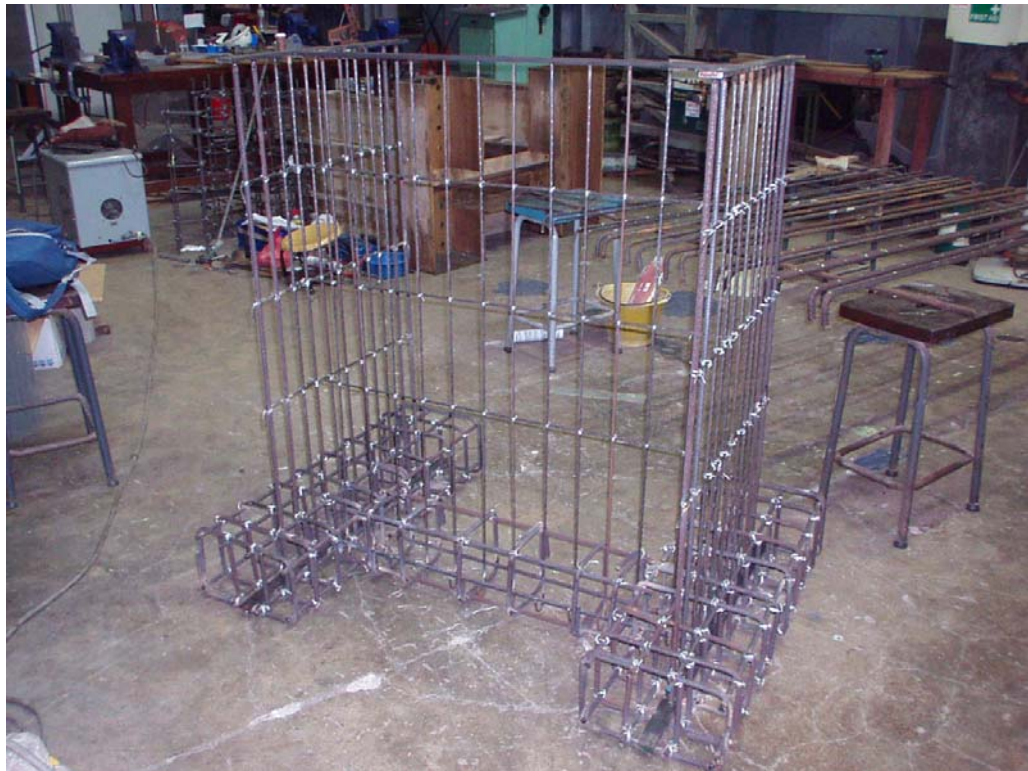
Figure 4.5 Overall 3D view of the rebar in the wall specimen
