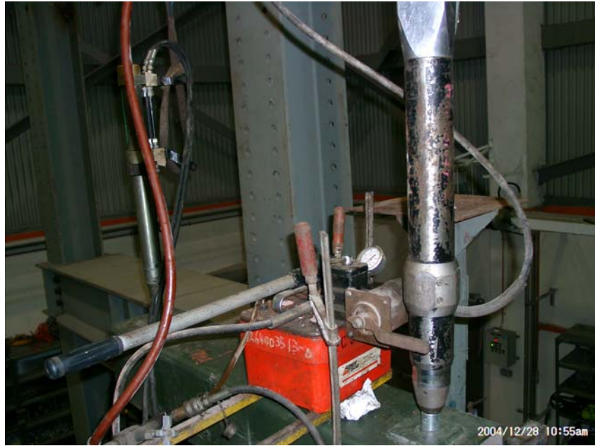
Figure 2.14 Two jacks were used together for one column
