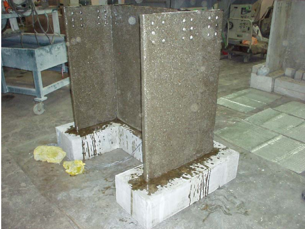
Figure 4.10 Wall after the application of MBT primer (Note the rounded edge of the wall)
