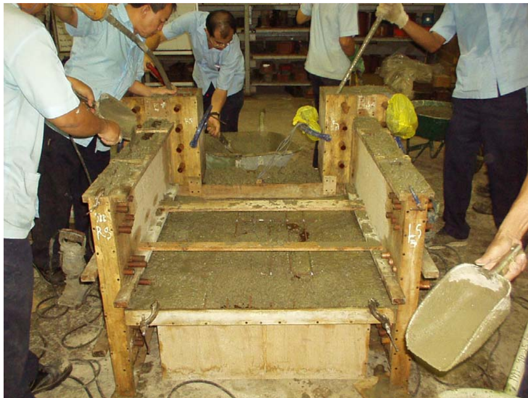
Figure 4.9 Concrete casting in the lab
