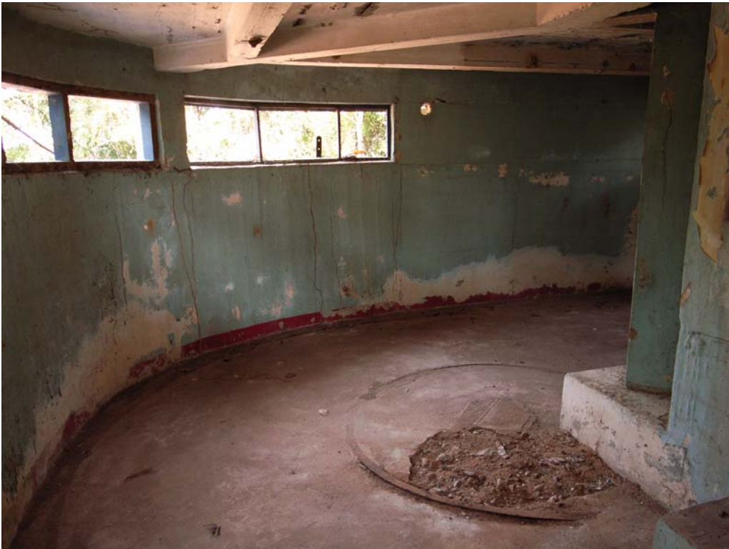
Illustration 81. Interior of the lower level of Connaught's BCP. (Aaron Kao)
