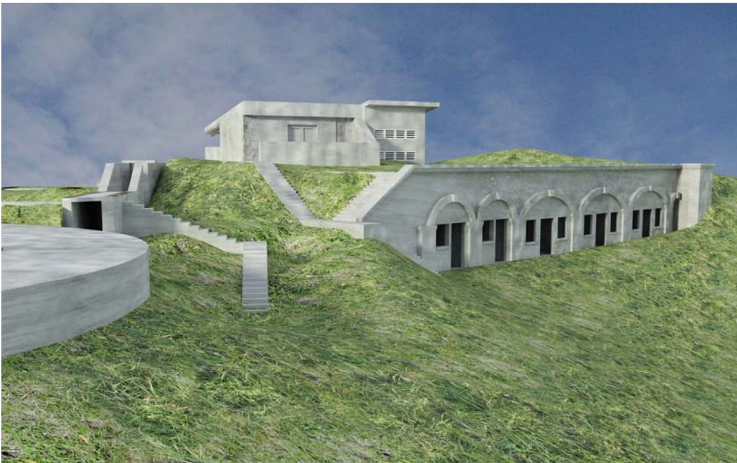
Illustration 29. Artist rendition of the Fort Serapong hilltop. (L to R) Apron of the 9.2 inch Gun No.2, followed by the communication trench, 9.2 inch BCP and annex, and casemates. (Daniel Hii)
