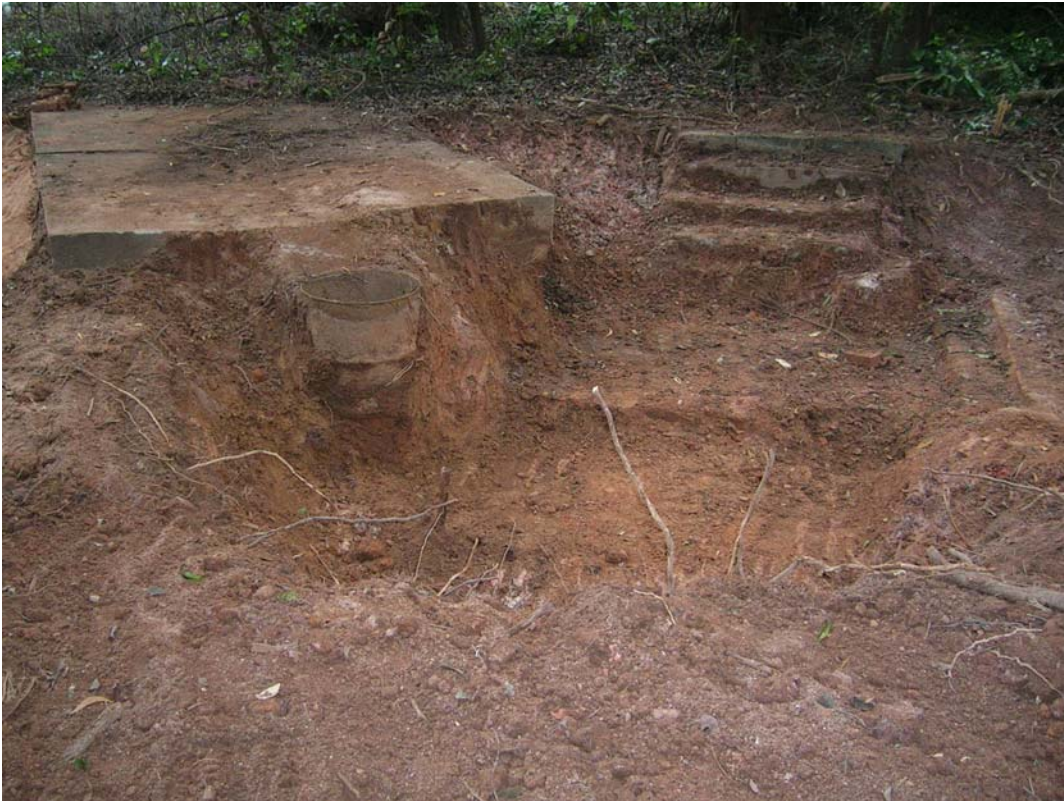
Illustration 98. Generator platform built over the old 8 inch Gun No.1 cartridge store. In front of the concrete slabs is the steel 55 gallon drum for collecting waste oil. (Author)
