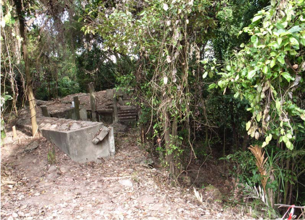
Illustration 60. The rear of 6 inch Gun No.2. To the right is the 30m wide crater where the magazine was formerly located. (Aaron Kao)
