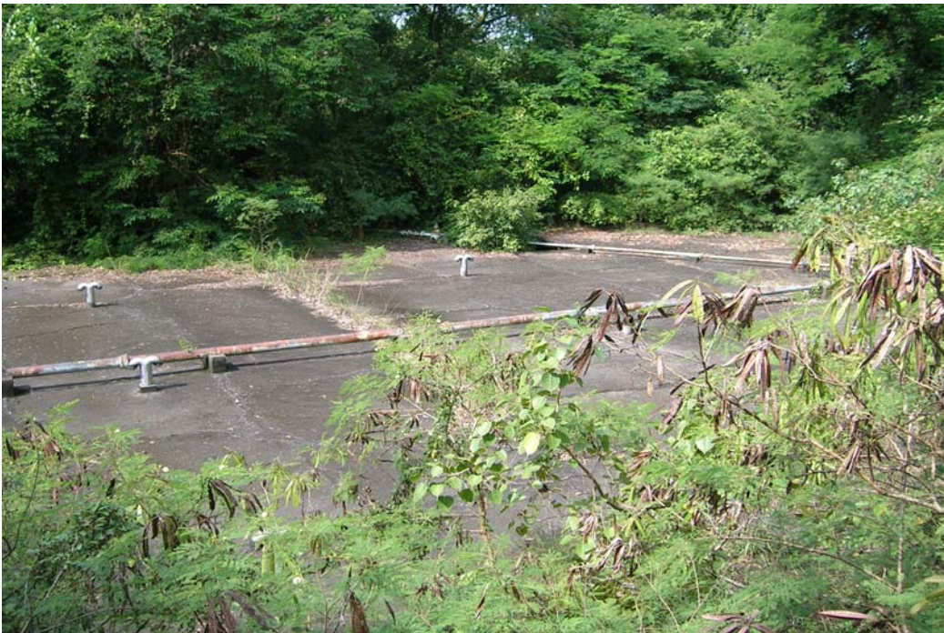
Illustration 41. The water storage tank because it was covered, led many researchers in the past to mistakenly identify it as an “underground” reservoir. (Author)
