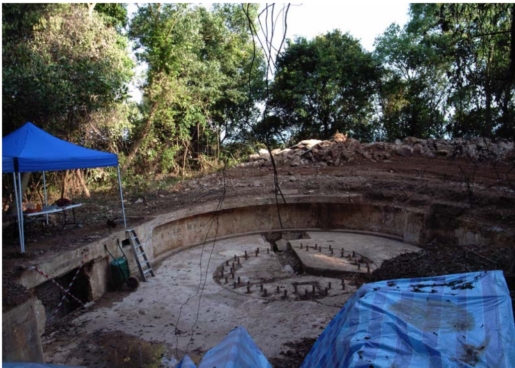
Illustration 27. View of the 9.2 inch Gun No.1 emplacement from the rooftop of Fort Connaught's battery command post. The accumulator pits and mounting bolts are clearly visible. Marked by caution tape on the left is the shell hoist. The curved recess beneath the parapet in front is for ready shells to be stocked. (Aaron Kao)
