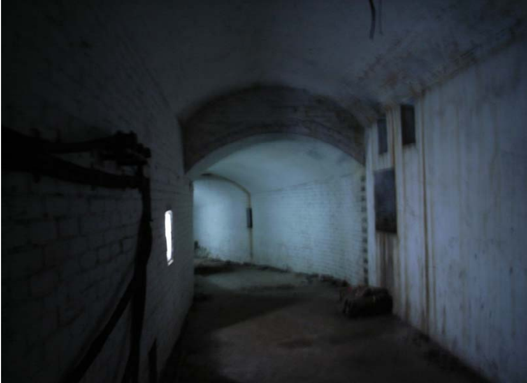
Illustration 32. 9.2 inch gun magazine and shell hoist passageway. The passageway ran on a north-south axis and lead to a shell hoist for the gun emplacements above at each end. Here looking north. (Aaron Kao)
