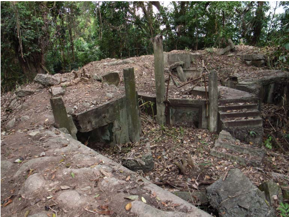
Illustration 55. 6 inch Gun No.2 Note concrete humps in foreground. (Aaron Kao)
