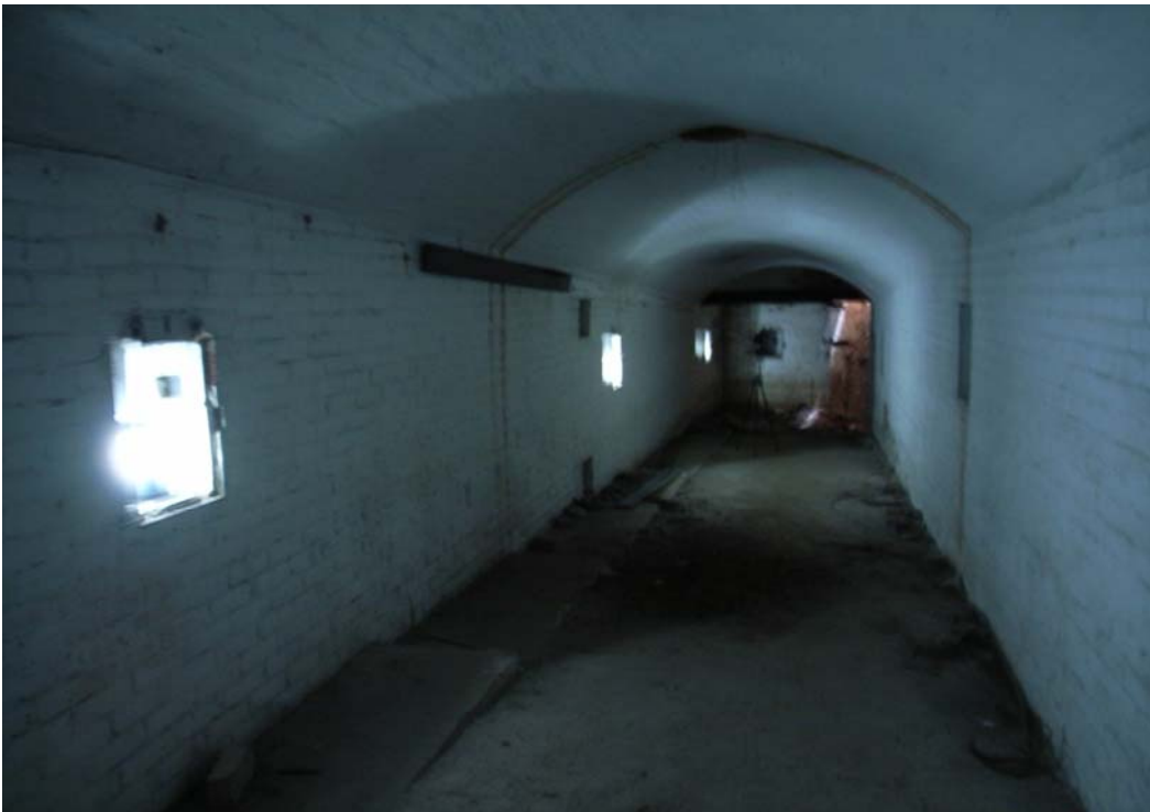
Illustration 33. Passageway looking south and towards the opening for the 9.2 inch Gun No.1's shell hoist at the end. The steps on the floor to the left are for timber skids for stacking the shells. (Aaron Kao)
