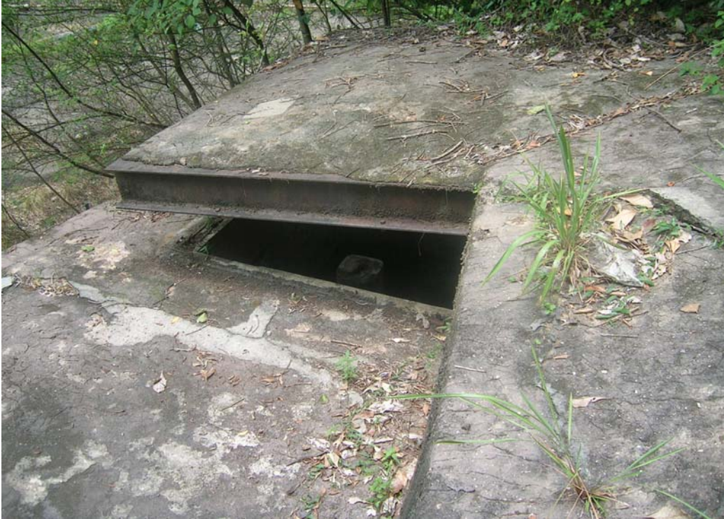
Illustration 42. PF Cell No.1 located on the southwestern edge of the watch catchment runoff. One of the concrete pedestals for range finding equipment is visible through the slit window. In the rear the water storage tanks can be seen. Unlike the other PF Cells, access was via a passage and stairs below at the water tanks. (Author)
