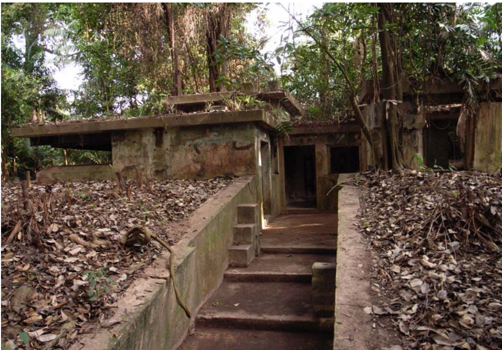
Illustration 69. Looking southwest, entry into the 6 inch gun BCP from the communication trench. On the left is the battery command post itself with the position finder. Straight ahead is the communications/radio room, and on the right is probably a large plotting or map room. Rising in the rear is the upper level of the BCP. (Aaron Kao)
