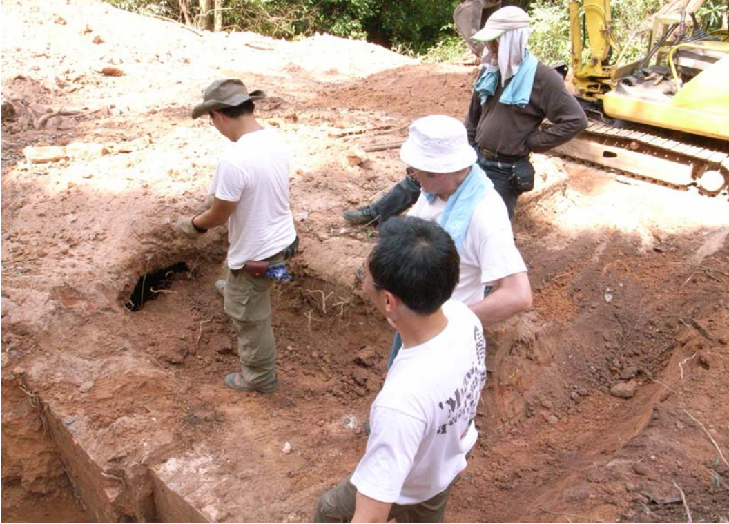
Illustration 5. The uncovering of the top of the 8 inch Gun No.2 cartridge store came as a surprise to the crew. (Aaron Kao)
