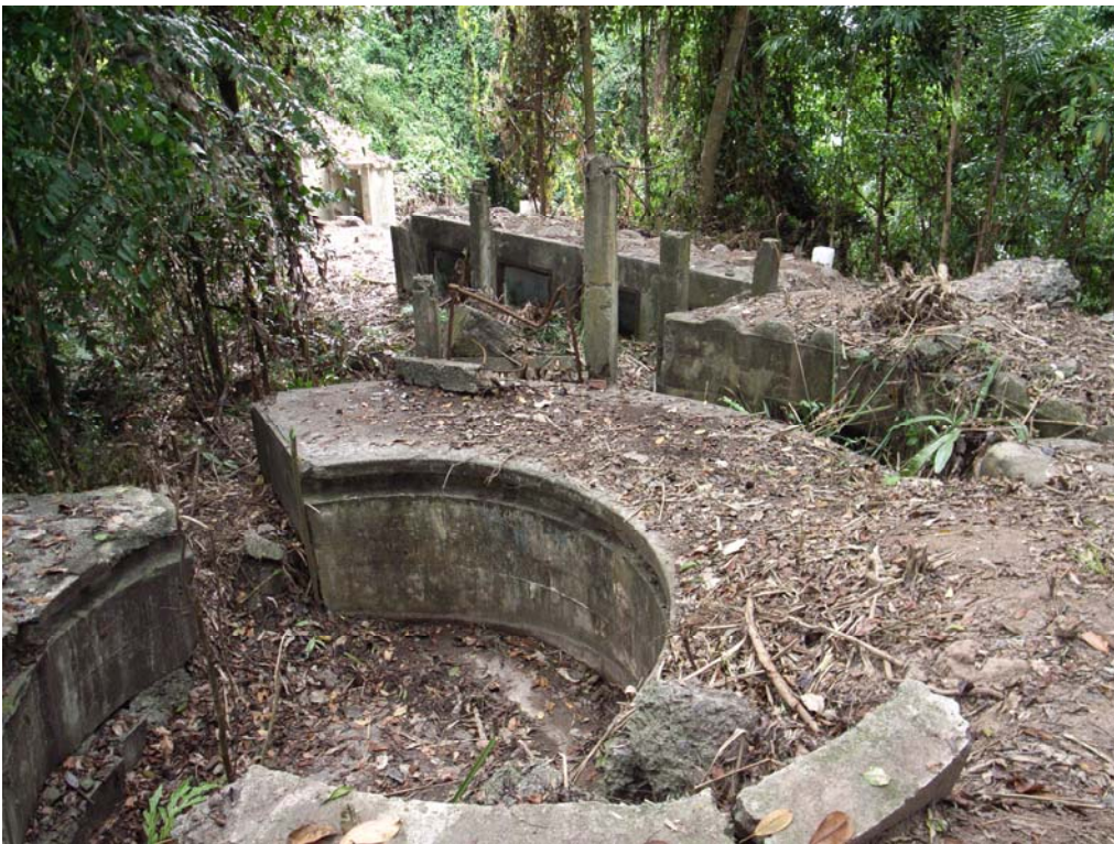
Illustration 57. Front view of the 6 inch Gun No.2 emplacement. The damage and shearing from the magazine's detonation is obvious. In the background under the sunlight is the gunners' shelter. (Aaron Kao)
