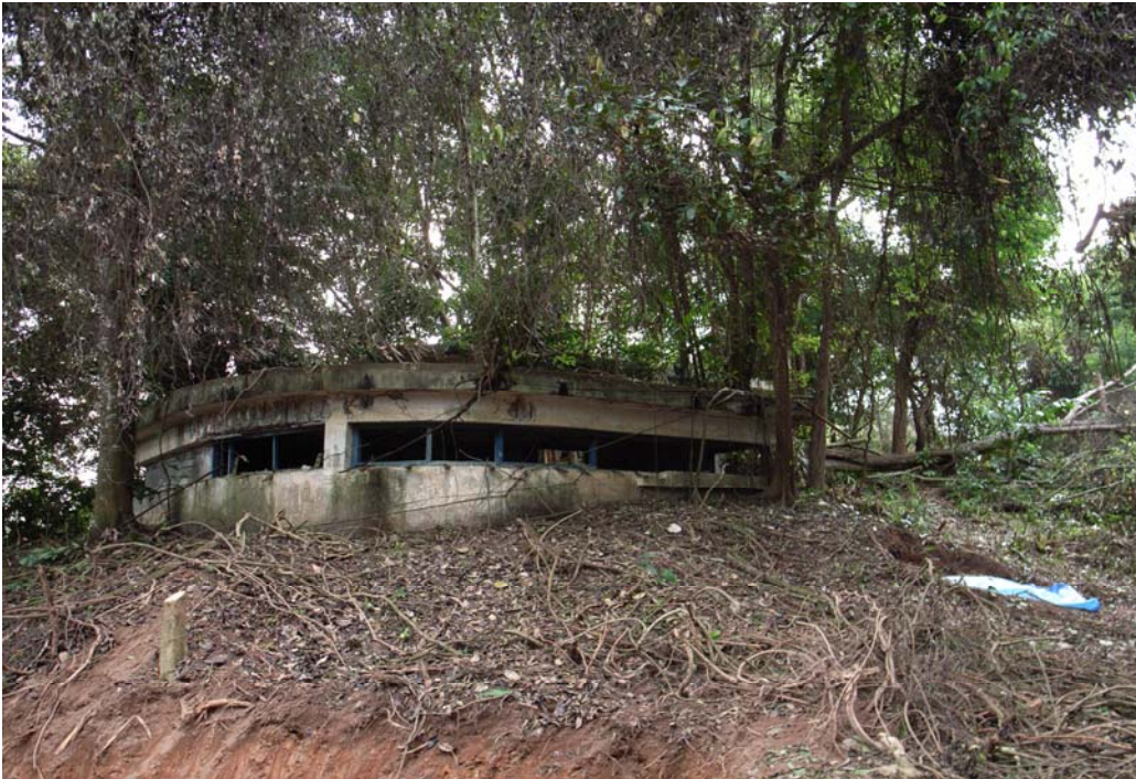
Illustration 79. Front view of Fort Connaught's BCP from the 9.2 inch Gun No.1 position. After the 9.2 inch guns were decommissioned and a new battery of 6 inch guns was built at the Spur, Connaught's BCP took over the hilltop of Mount Serapong. (Aaron Kao)
