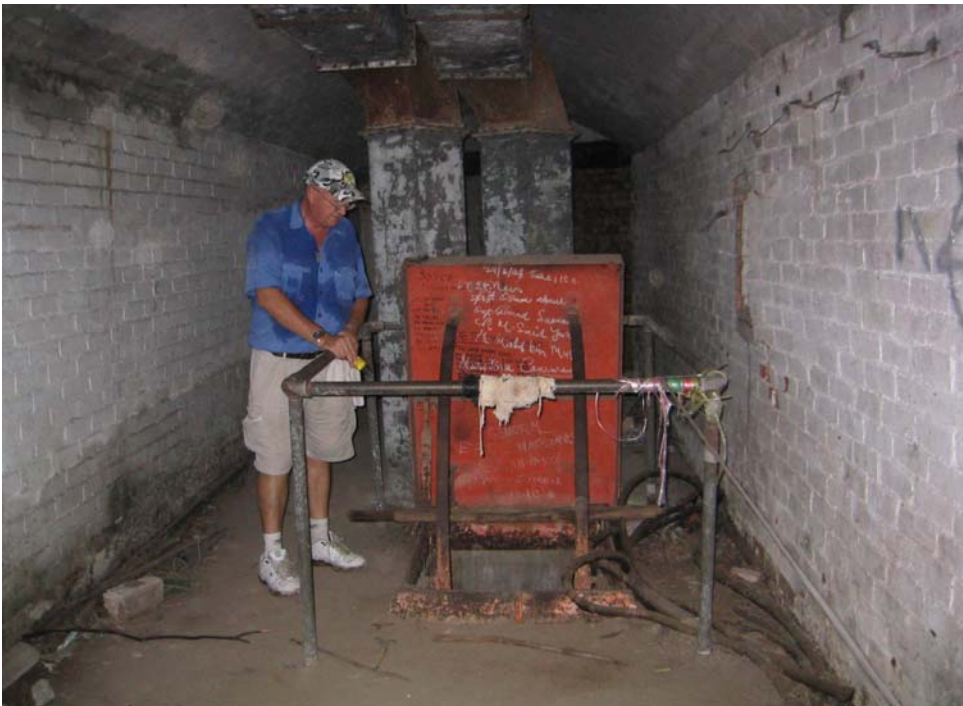
Illustration 86. Derek Potter looks down into the escape shaft, 17m above from the 9.2 inch magazine passageway. Note ventilation ducts for command centre in rear. (Author)
