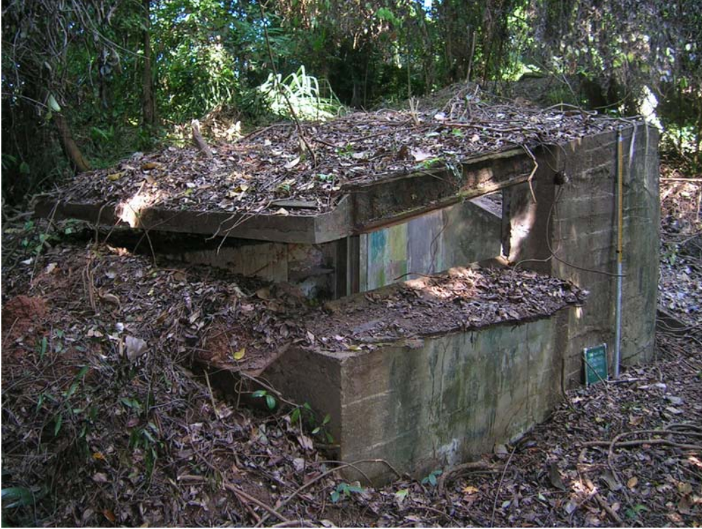
Illustration 18. PF Cell No.7 was one of the four cells which remained today on Mount Serapong. At one point in time there were a total of seven such structures. (Author)
