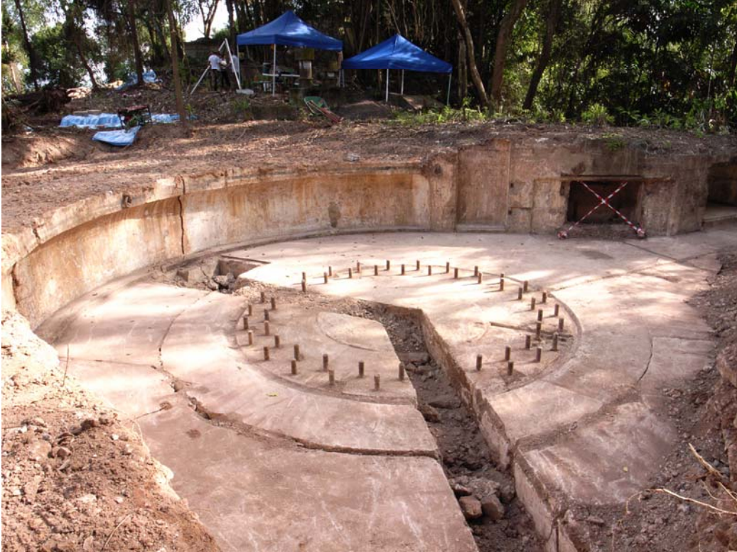
Illustration 30. 9.2 inch Gun No.2 emplacement with its accumulator pit and trench prominently exposed. In the background wrapped by the banyan tree is the battery command post. Gun No.1 is beyond the little rise out of sight on the top left corner of the photograph. (Author)
