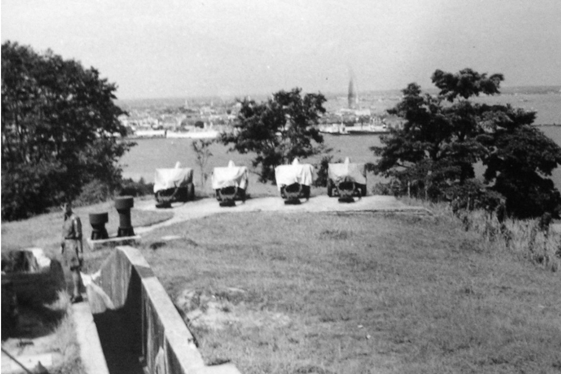
Illustration 105. Post war saluting battery atop Mount Serapong. The concrete platform is erected over the old 9.2 inch Gun No.2 emplacement. The soldier is standing over the old communication trench and midden. (Author's Collection)
