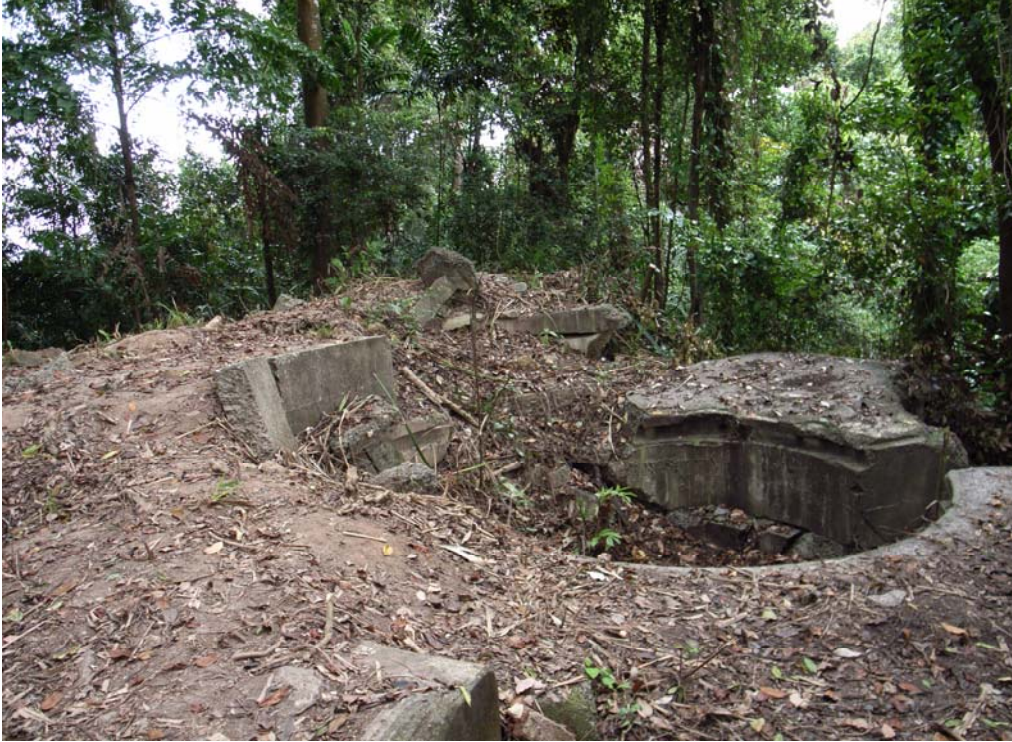
Illustration 58. Another view showing damage from magazine explosion. (Aaron Kao)
