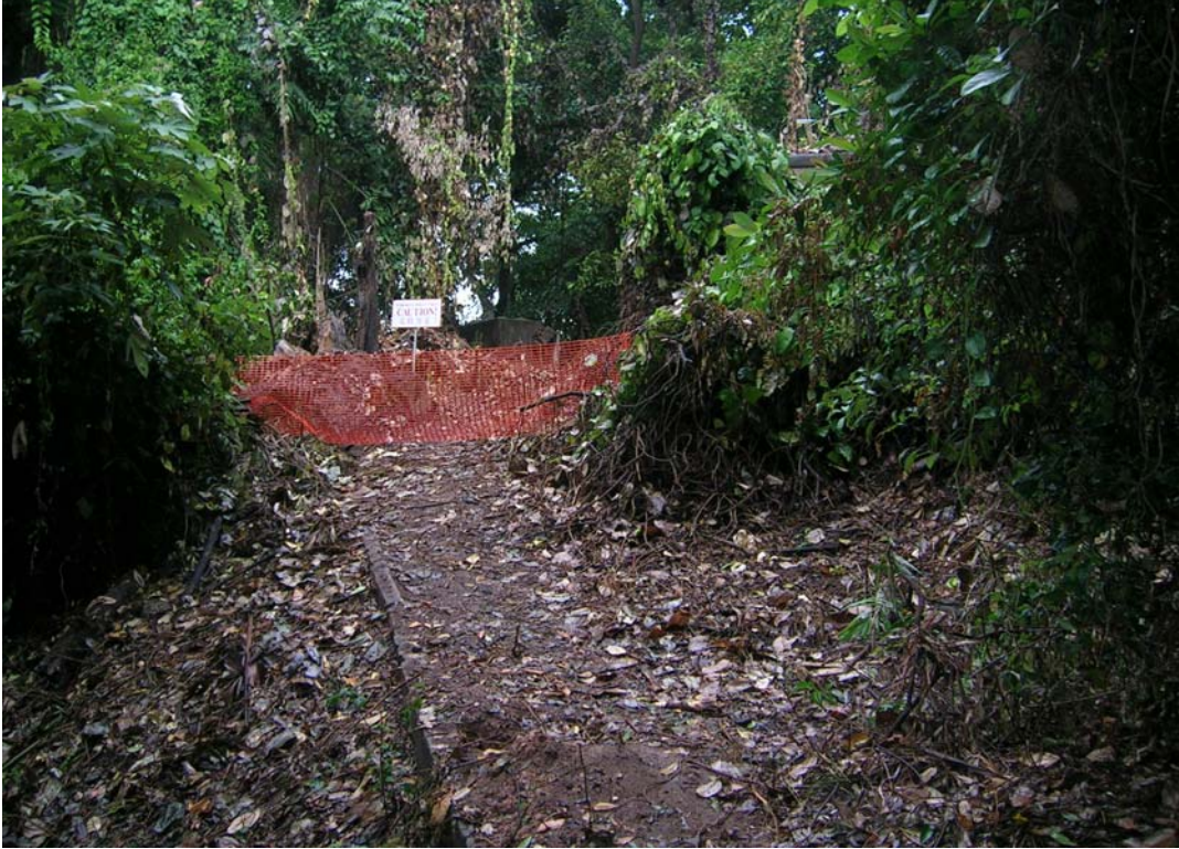
Illustration 66. Concrete and gravel ramp leading to the 6 inch Gun No.2 position from the road. The gunners' shelter is on the top right hidden by the vegetation. (Aaron Kao)
