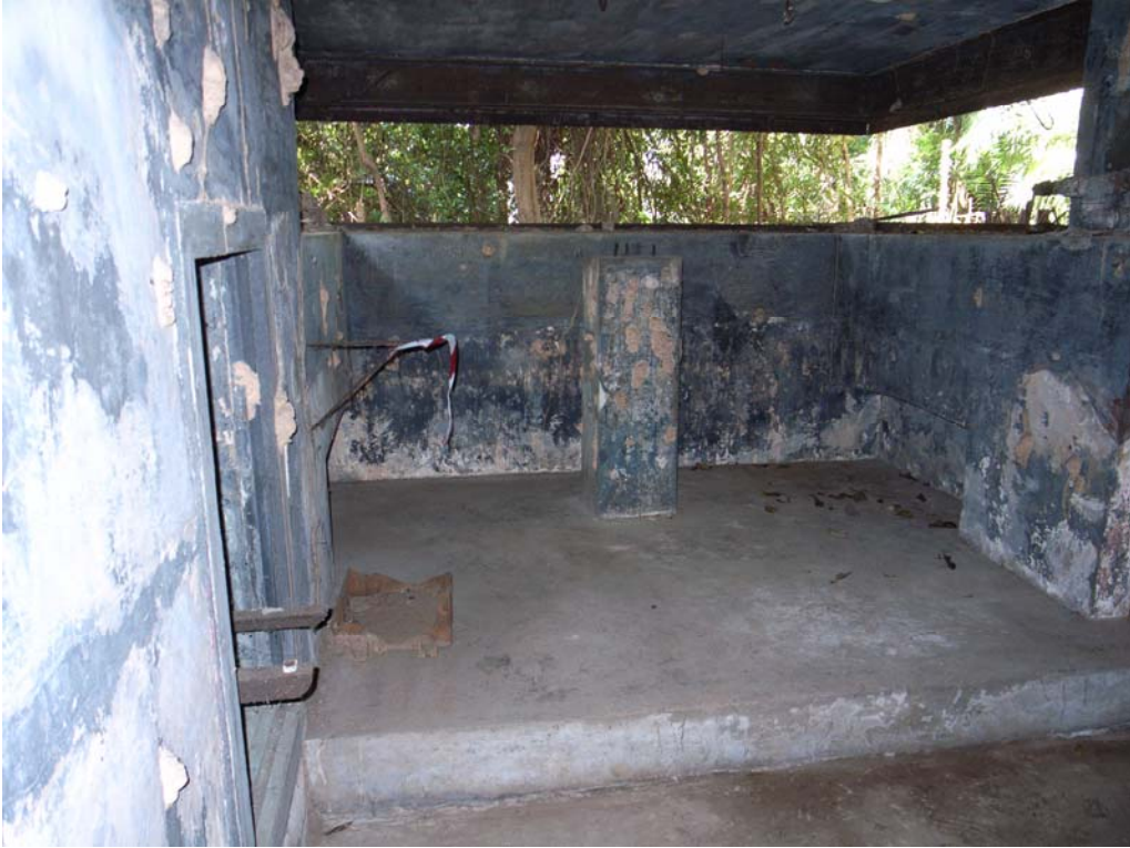
Illustration 70. Interior of the 6 inch gun BCP lower level. A single pedestal mount with bearings and instructions painted on is still in situ. (Aaron Kao)
