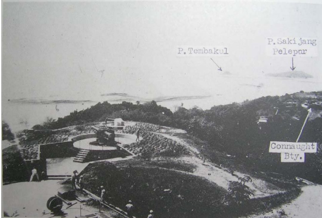
Illustration 92. The only known photograph showing the Serapong Spur Battery pre-Second World War. The pair of 6 inch guns laid out in tandem is clearly depicted. At the time when the photograph was taken, the overhead canopies have not yet been installed. (National Archives United Kingdom)
