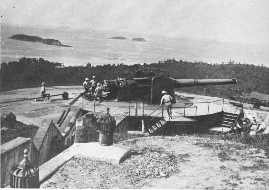
Illustration 28. The 9.2 inch Gun No.1 in its heyday. Several gunners could be seen sheltering in the shade of the communication trench to the left. In the foreground were two Howorth's revolving ventilators for the magazine below. In the distance, were the islands of (L to R) Pulau Sakijang Pelepah (Lazarus), Pulau Sakijang Bendera (St.John's), Pulau Sabar Laut, and Pulau Subar Barata (Sisters Islands). (Author's Collection)
