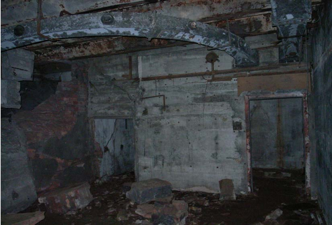
Illustration 83. Interior of the main room of Blakang Mati command centre. The doorway leads to a smaller room where the air purification plant was located. Note intake and output air ducts above. (Author)
