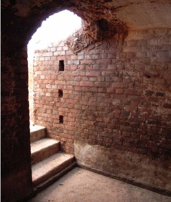
Illustration 7. Interior view of the 8 inch Gun No.2 cartridge store. (Aaron Kao)
