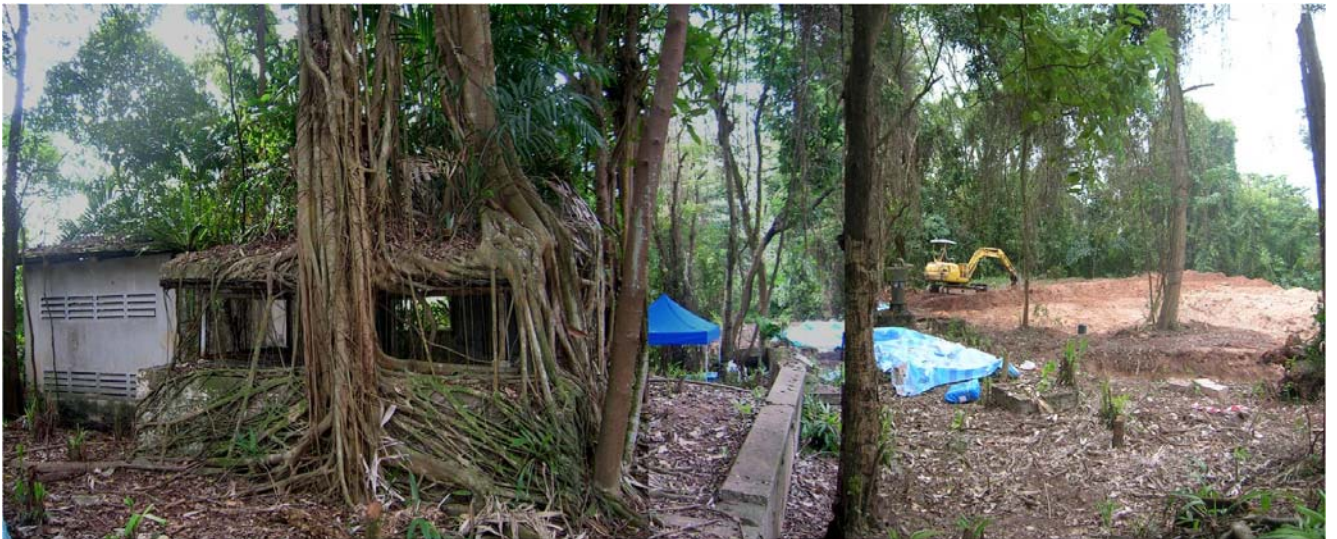
Illustration 31. 9.2 inch gun BCP (enveloped by banyan tree). On the left is the annex building added on at a later date with its ventilation grilles clearly visible. The concrete wall (centre) is part of the communication trench connecting the two gun positions. Gun No.2 is to the right where the excavator is pictured. The BCP overlooks Gun No.1. (Author)
