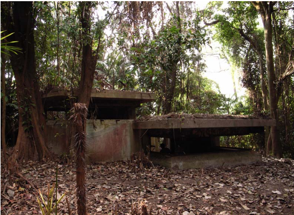
Illustration 71. Front view of the 6 inch gun BCP. The structure is split leveled with the lower room built into the earth and the upper room at ground level. (Aaron Kao)
