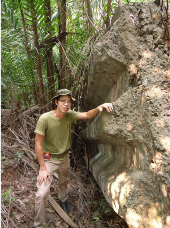
Illustration 61. Aaron Kao provides a scale to the massive block of concrete that was once the roof of the magazine. (Author)
