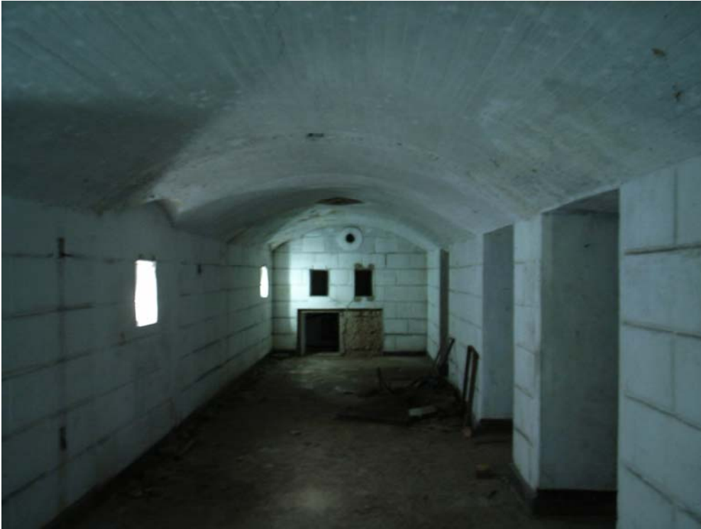
Illustration 13. 8 inch gun magazine shell and cartridge store as seen today. The cartridge store would have been the front half of this chamber and separated by a wall since removed. Modern lanterns glow in the lamp recesses. (Aaron Kao)
