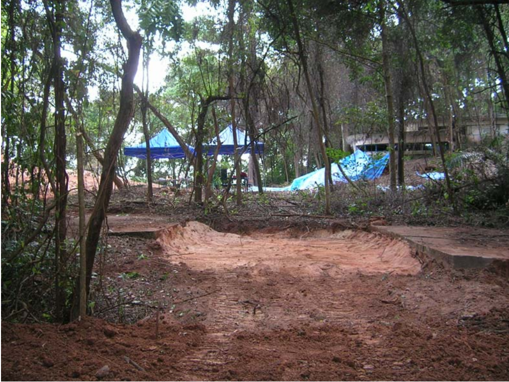
Illustration 99. The pair of generator platforms. Visible in the rear just beyond the tents is the 9.2 inch Gun No.1 emplacement. To the right is Fort Connaught's BCP. (Author)
