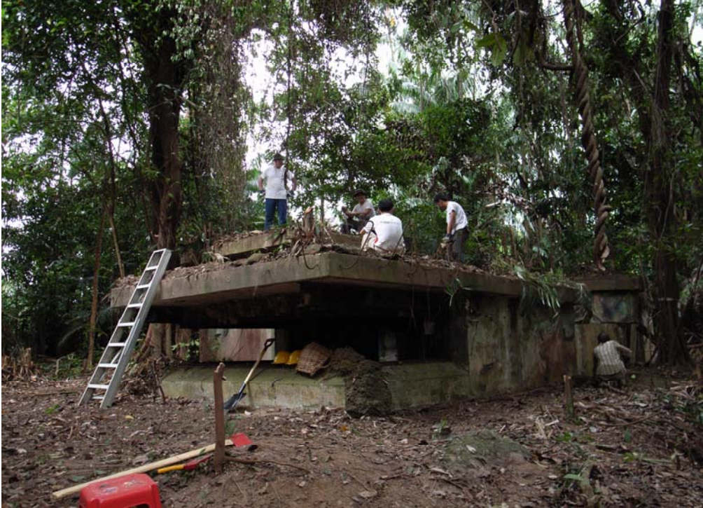
Illustration 68. Field crew working on the BCP's rooftop. Hooks for camouflage netting are still in place along the edge of the roof. (Aaron Kao)
