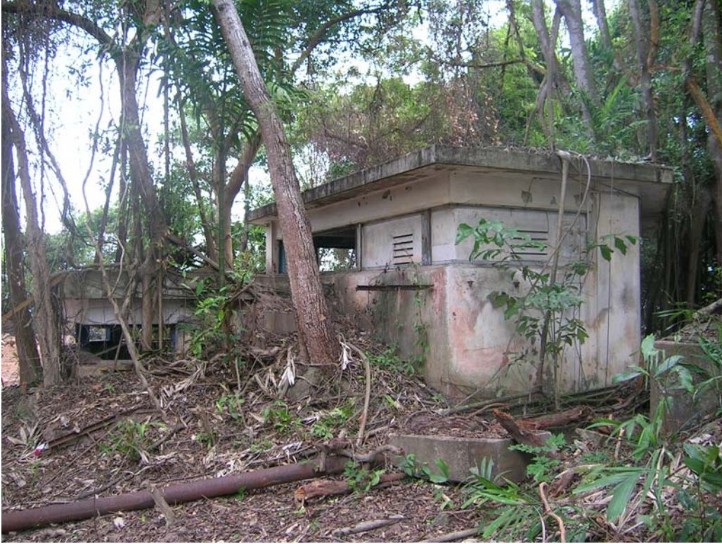
Illustration 82. Connaught's BCP as seen from the rear. To the right in the foreground are remains of the 9.2 inch gun communication trench. (Aaron Kao)
