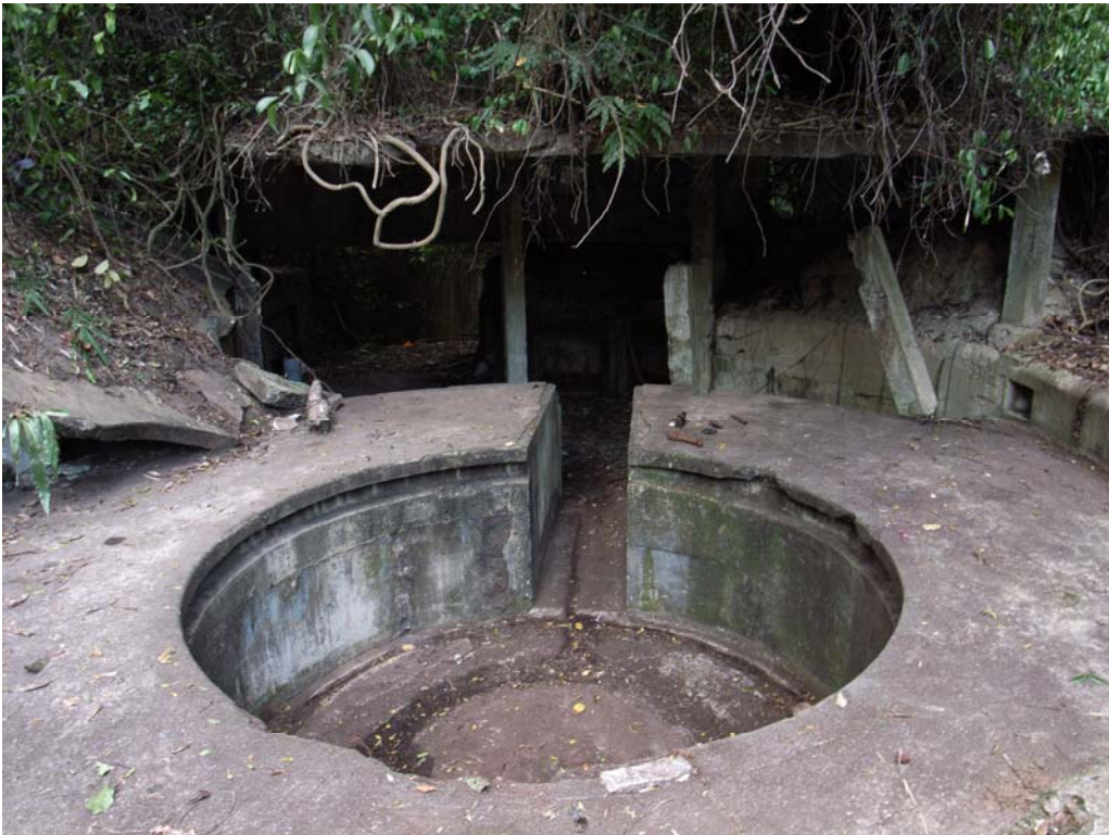
Illustration 47. The same gun position after removal of the jungle growth. Traces of the older 9.2 inch gun parapet can still be seen on the right encircling the smaller 6 inch gun carriage well. (Aaron Kao)
