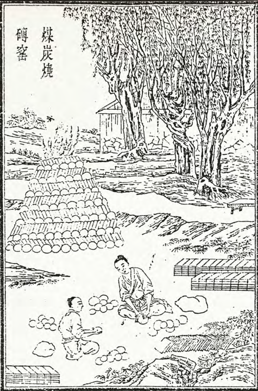
A brick kiln-- coal is used as the main fuel.
