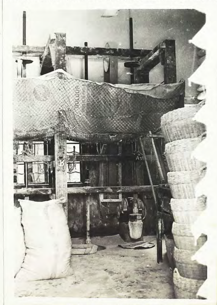
A modern machine for hulling rice, driven by a motor.
