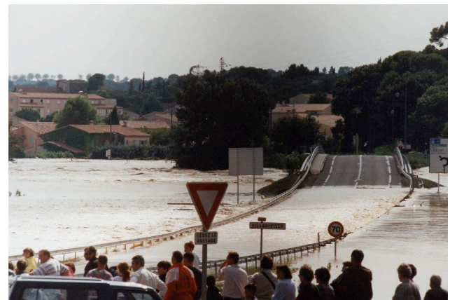
Fig. 8. Example of a submerged access road to the river crossing structure located in the flood plain (Gard 2002 flood upstream the town of Sommières).
