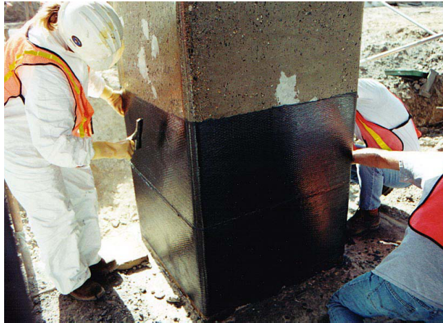
Figure I.2. 6: Confinement de colonnes (Pantelides et al. 2002)
