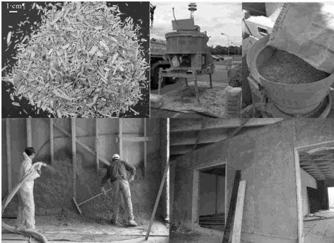
Figure 1. Hemp concrete Spaying Method: the mixer / lime and vegetable particles mixing / spraying.
