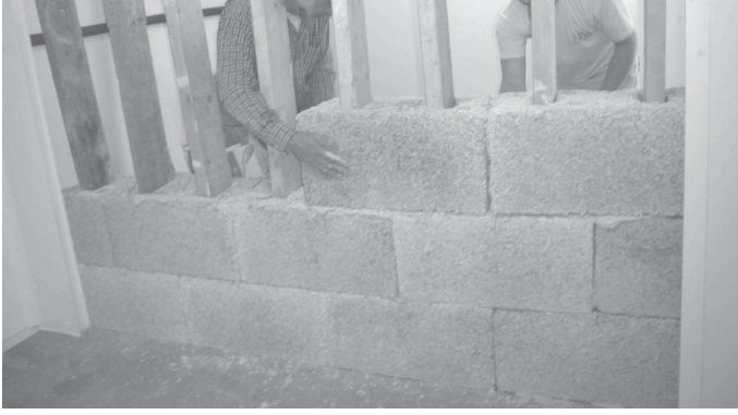
Figure 4. Building of the test wall
