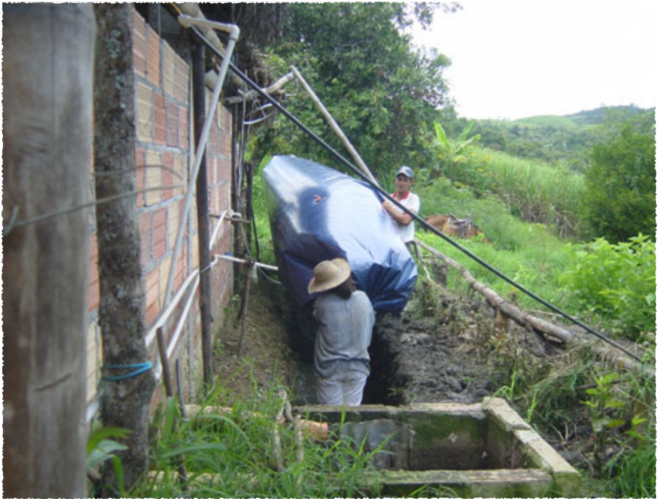
Placing the biodigester in the trench.
