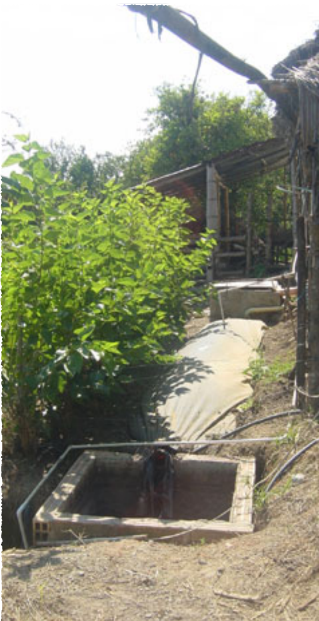
Biodigester made with one layer of plastic of 1.2 m diameter and 6 m long, connected to a pig pen with 20 animals and fenced with Mulberry tree. Finca Ecológica Tosoly, UTA Foundation, Guapotá, Santander, Colombia.
