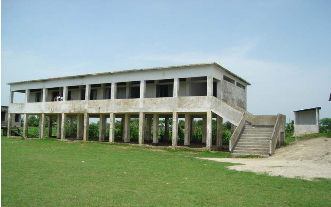
Figure-24: A Multi-purpose Cyclone Shelter, Where the Only Toilet is Located Outside
