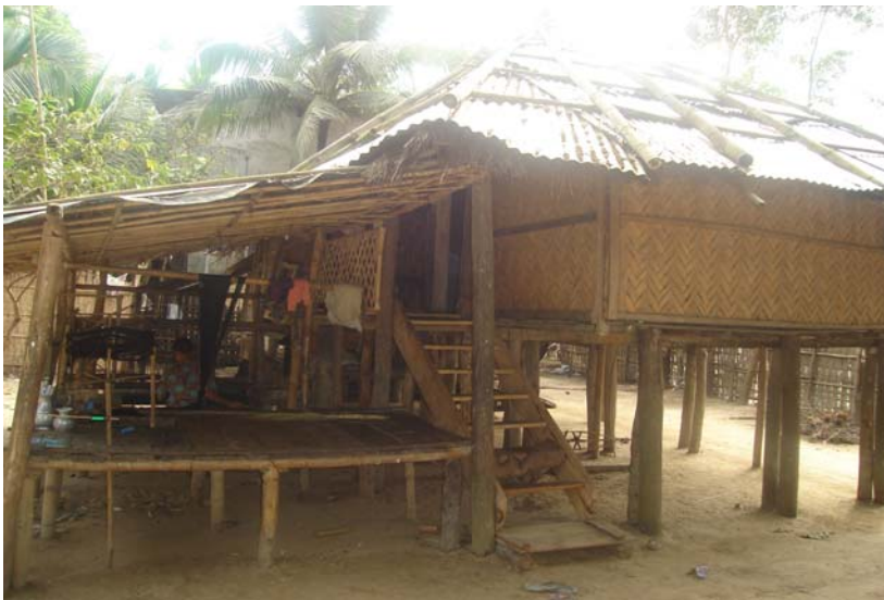
Figure-22: House built on stilts – an example of coping practices
