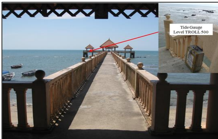
Figure 3.22 The tidal station at Tg. Balau jetty
