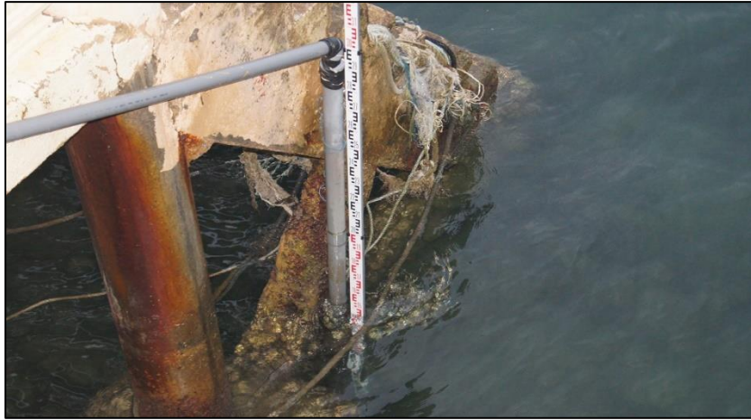
Figure 3.23 Manual checking for tidal elevation at Tg. Balau Jetty
