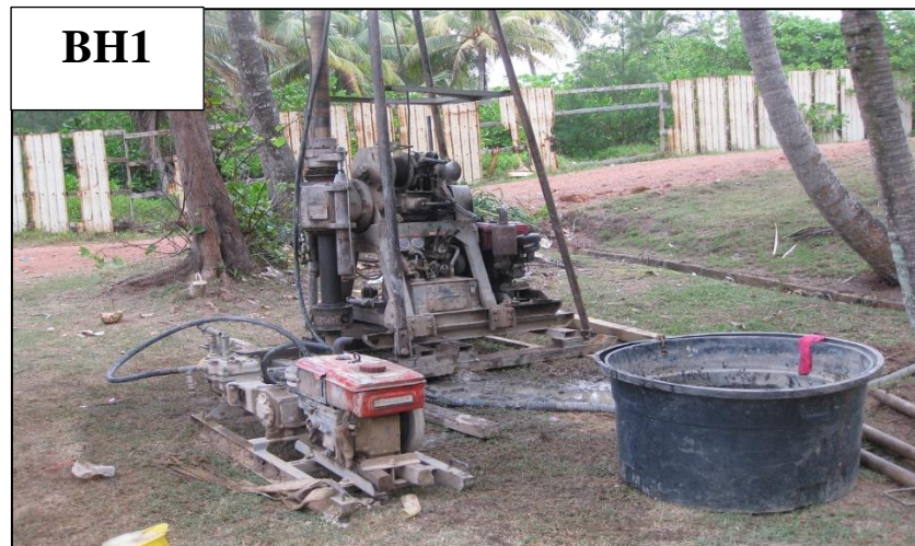
Figure 3.12 Boring and drilling pump of well BH1
