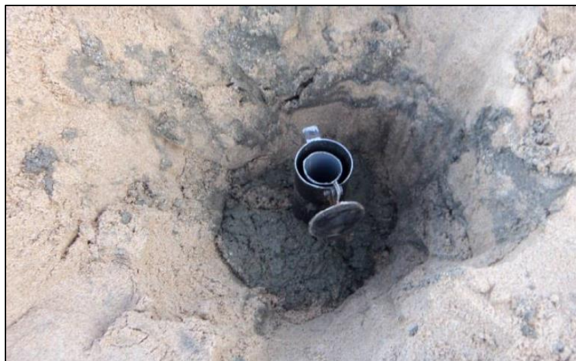
Figure 3.16 The concrete cement is placed at the top of borehole
