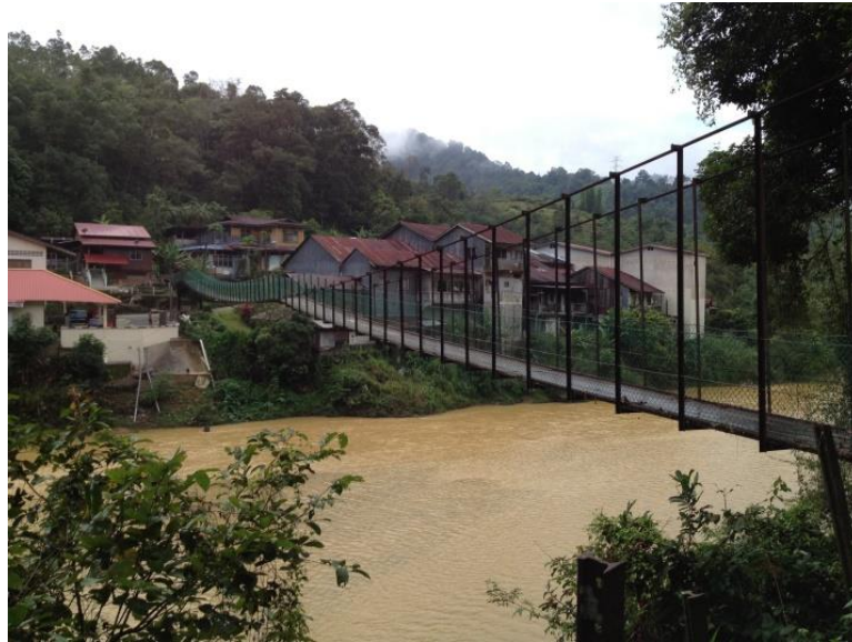
Figure 5. Kolong Pahat hanging bridge.
