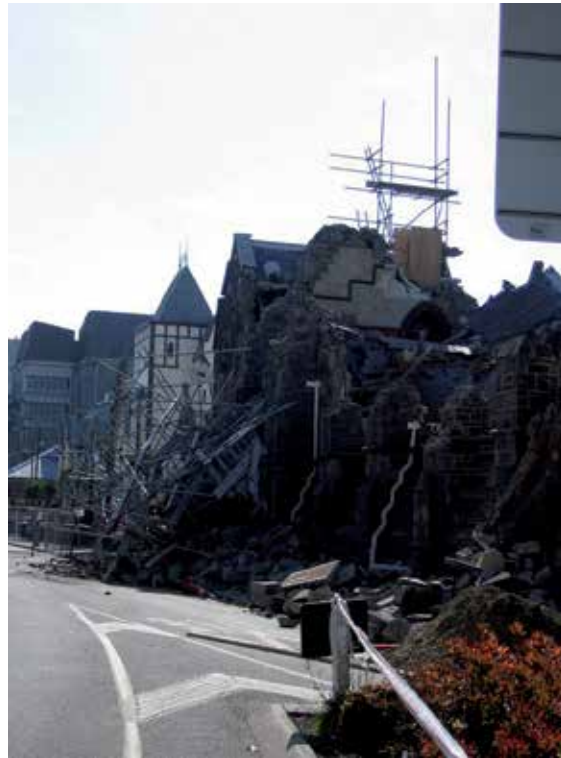
Figure 7. Canterbury provincial buildings post-earthquake [Diane Brand] 2011
