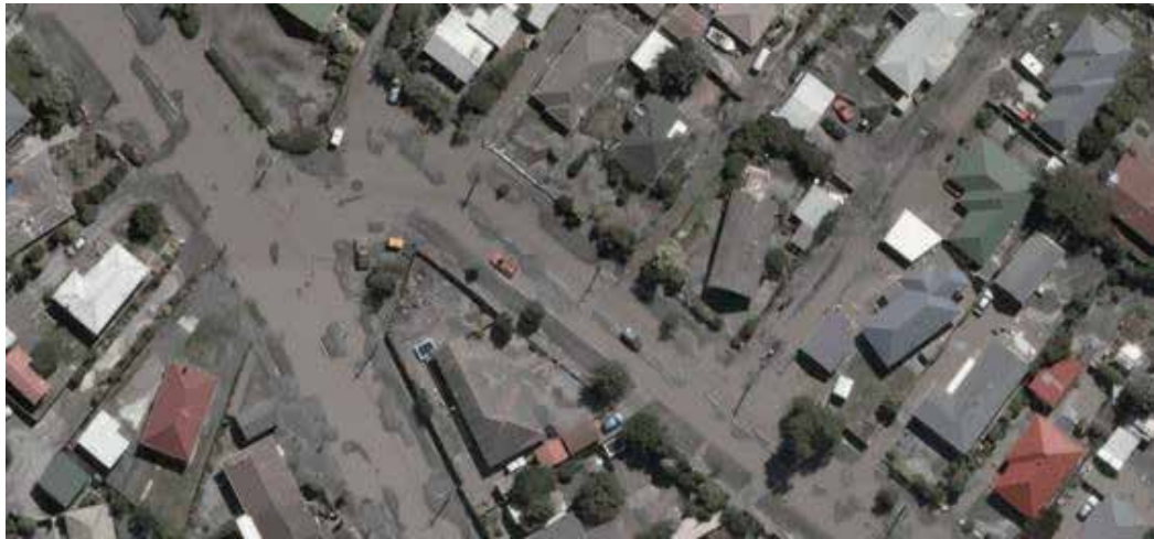
Figure 8. Liquefaction in the eastern suburbs of Christchurch (2011) New Zealand Aerial Mapping Ltd for LINZ
