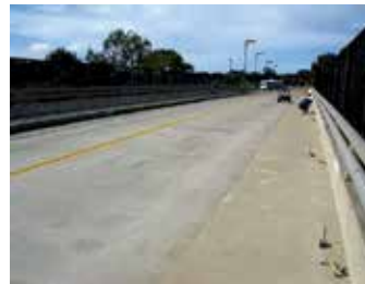
(c) Side view of the bridge over Interstate 5
