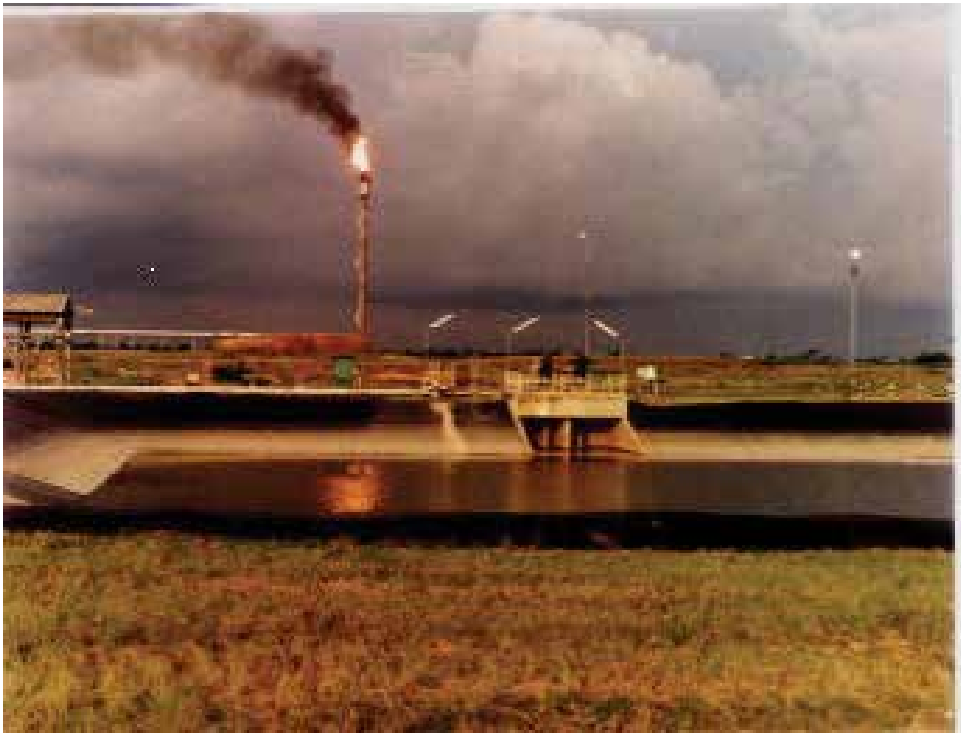
Plate 4. Emissions from a Petrochemical plant
