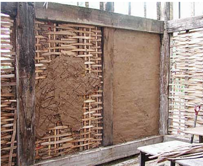
Figure 10: Timber-framed building with panels at various stages of wattle & daub infill [17]
