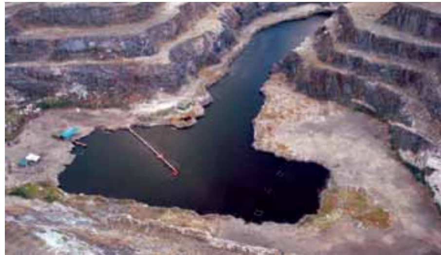
The lake formed when a tin mine eventually dug into an underground aquifer.
