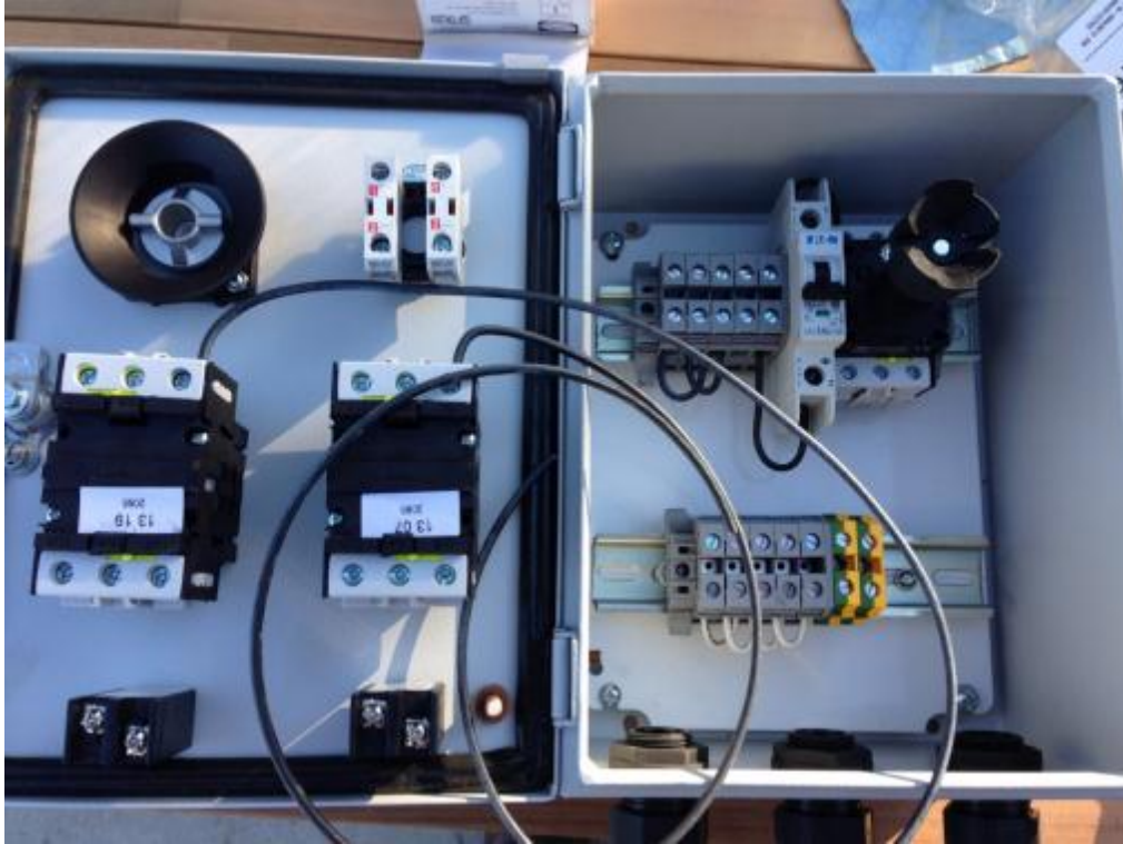
Figure 57 : Nearly Complete Electrical Box
