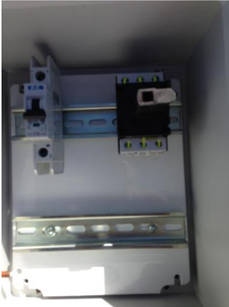
Figure 56 : Installation of DIN Rails
