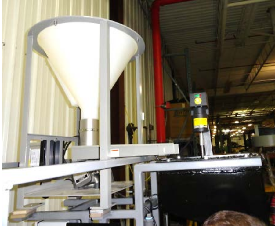
Figure 30: The Vibrating Feeder Moves Material into the Hopper
