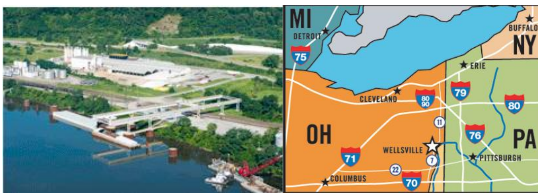
Figure 25: Wellsville Intermodal Terminal (Wellsville Terminal Co., 2014; O'Brien, 2013)
