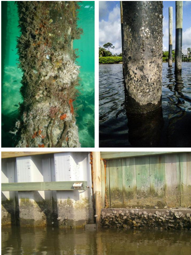
Figure 2. (a) A wood piling near Jupiter Inlet supporting a diverse community of filter feeding organisms. (b) Pile wrap material prevents colonization of most filter feeders. (c) Dock pilings are just one artificial substrate in urbanized coastal systems, with bulkheads being another common shoreline type. Note the distinct differences in fouling communities among bulkhead types.
