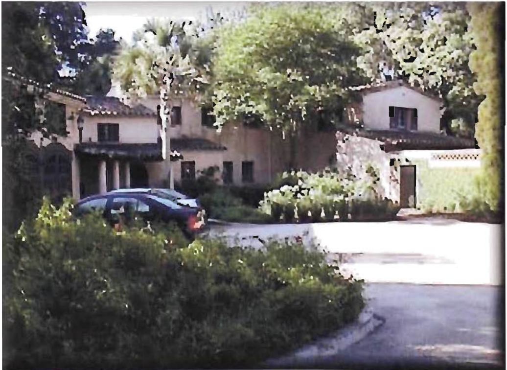
Figure 5.4 - Service entrance with handicapped parking area Source: Photograph by the author
