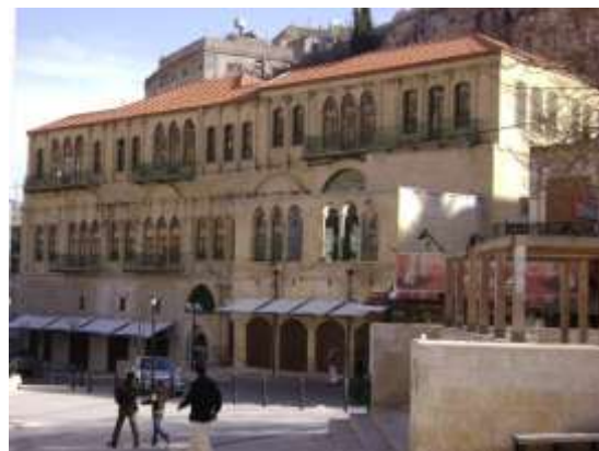
Figure (6.8): Abu Jaber Building (Al Salt Traditional Museum).
