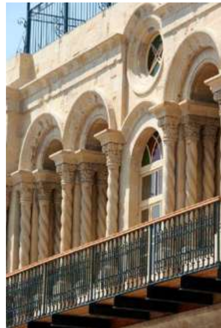
Figure (6.5): Muasher Building (Main Façade). Source: Researcher, 2010
