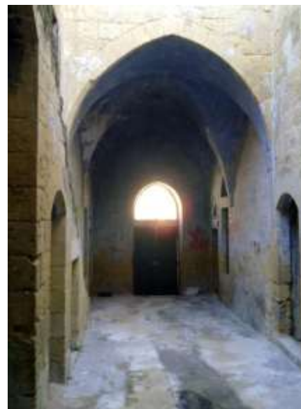
Figure (7.13): Open-sky-light Court of the Al-Khateeb Building Source: Researcher, 2010
