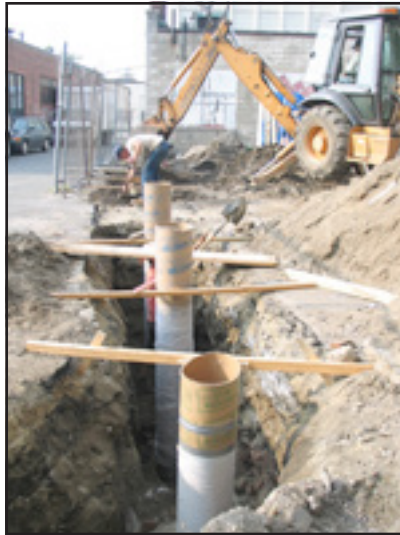
Figure 7: Foundation below freeze line
