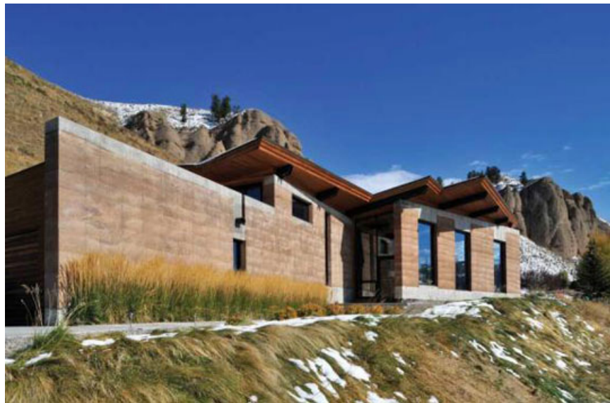
Figure 5: A modern rammed earth house in Wyoming
