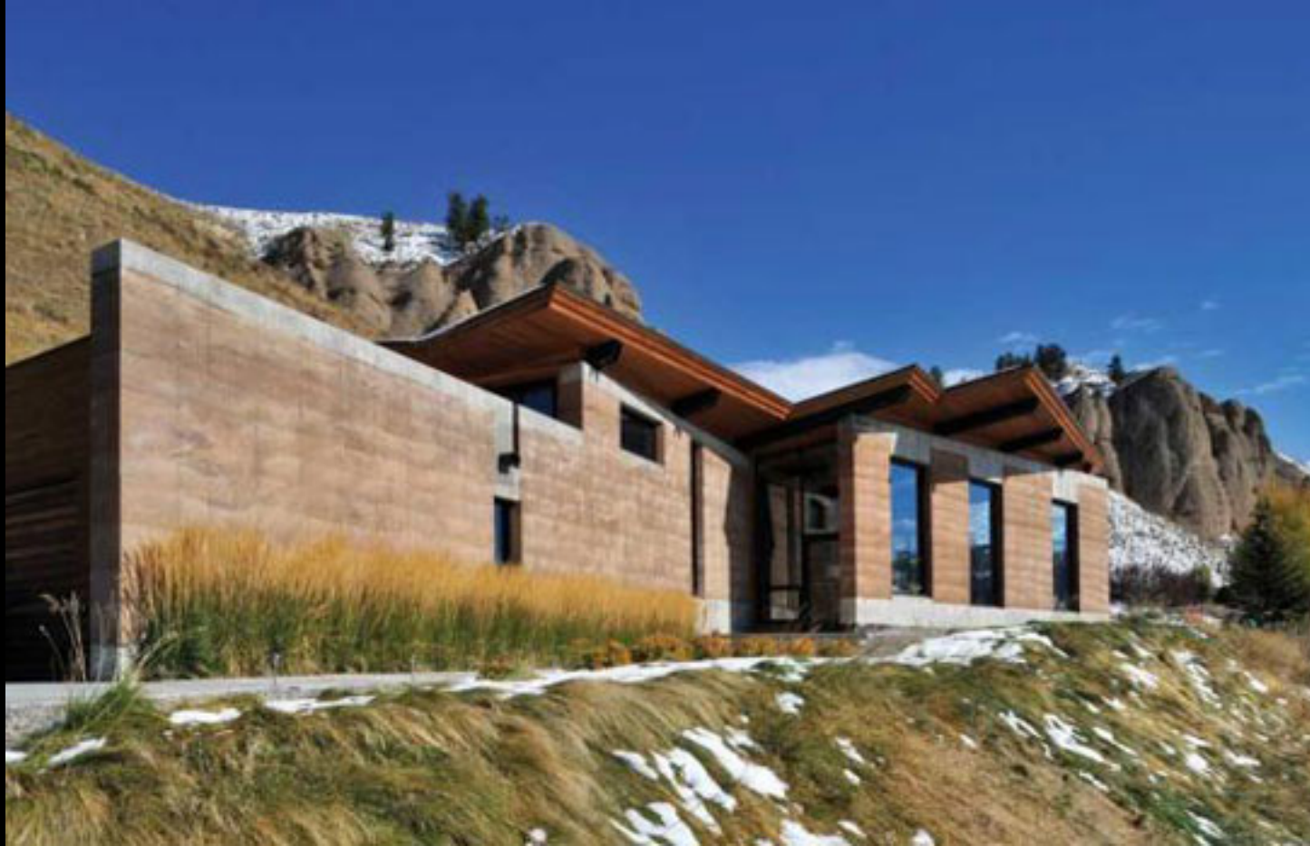
rammed earth construction
