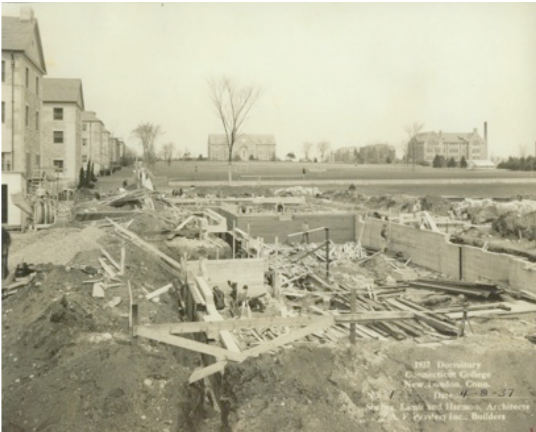
Figure 50. The construction of Freeman House, pictured above in its early stages, caps the line of student residences defining the west side of the Campus Green. Photograph, 1937.
