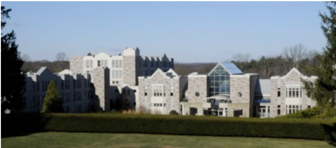
Figure 84. North Complex after the refurbishment of the 1990s, which stripped the buildings of their Modernist forms. Photograph by Lisa Brownell, 2000.
