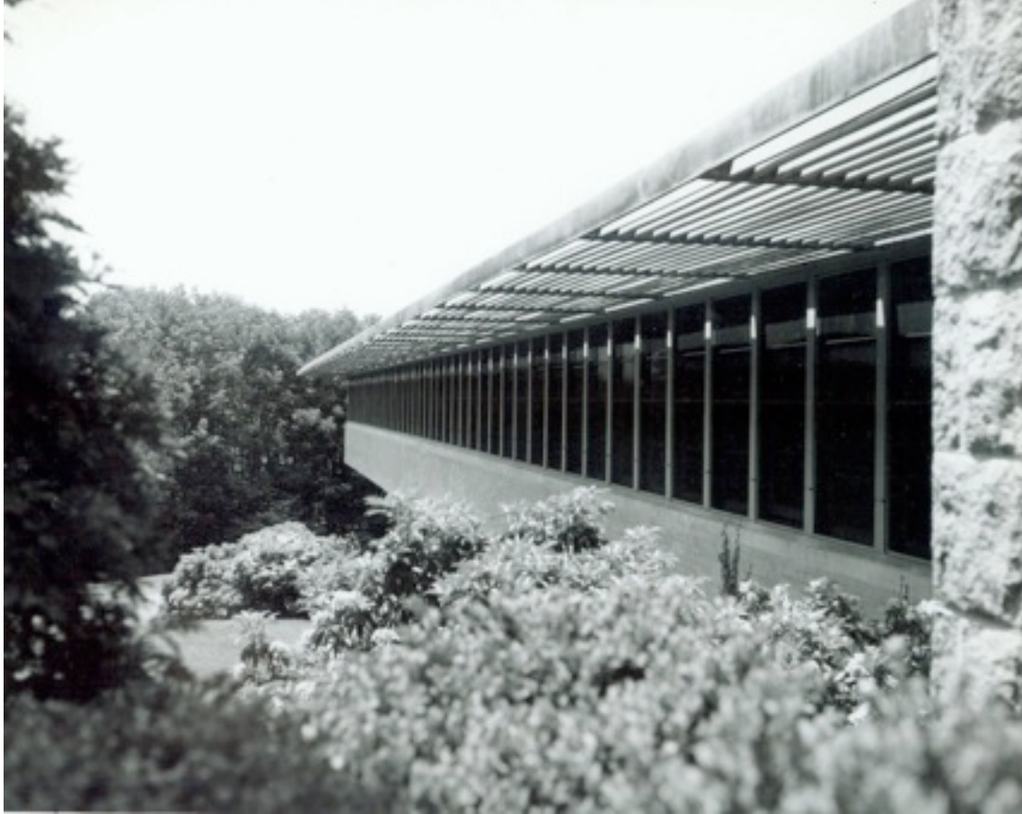
Figure 67. With its dramatic cantilever and unadorned facades, Warnshuis Infirmary was the first truly modern structure on the campus. Photograph, 1951.
