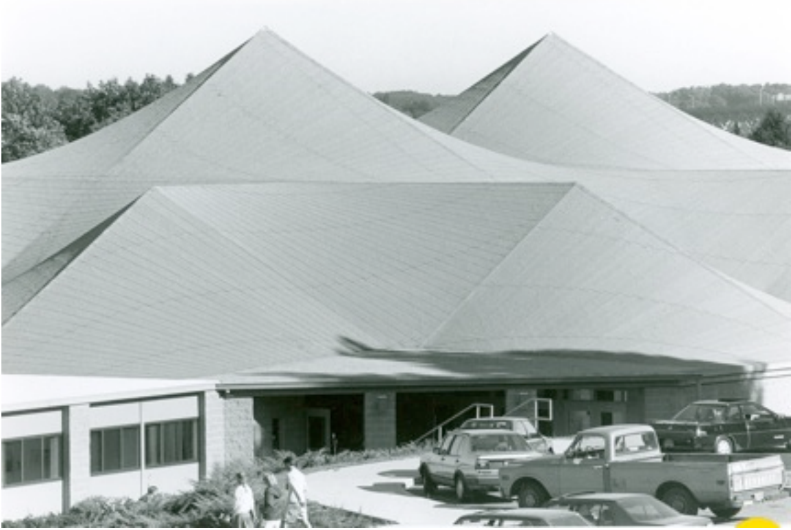
Figure 95. The parabolic roof structure of the athletic complex allowed for both efficient construction and a signature design. Photograph, 1986.
