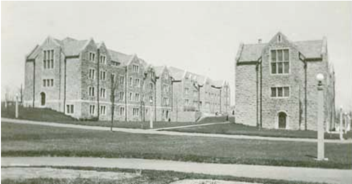
Figure 14. Three residence halls, Blackstone House, Plant House, and Branford House, were constructed in keeping with the Ewing and Chappell plan. Postcard, 1920.
