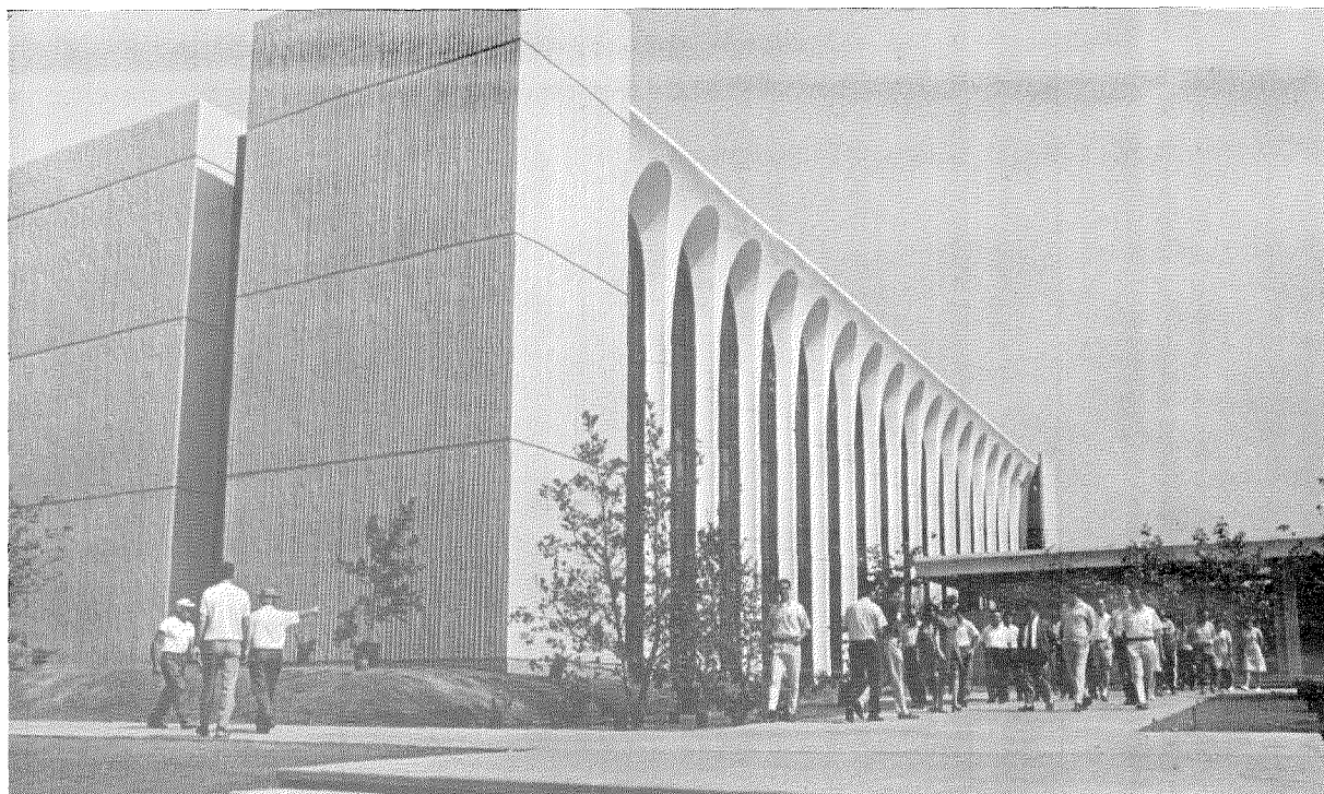
The new Noyes Laboratory—five stories, 90,000 square feet of offices, laboratories, and workrooms—was made possible by a gift from an anonymous alumnus and matching funds from the National Science Foundation.
