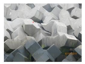
Figure 1.3: Broken Armour Units on breakwater (picture courtesy Royal HaskoningDHV)
