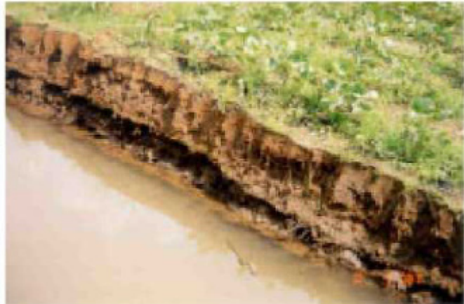
Figure 1.1: Erosion of a bank of the Mekong, Vietnam (from Le Viet Dung et al (2003))
