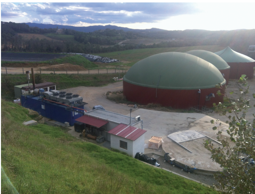
Figure 6.6.1. General view of Apergas treatment plant in Vilademuls (Catalonia, Spain).
