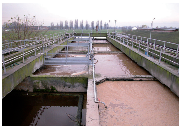
Figure 5.4.3. Aerobic process with aeration (left) and anoxic phase (right) in different tanks. In the foreground the sedimentation tank.
