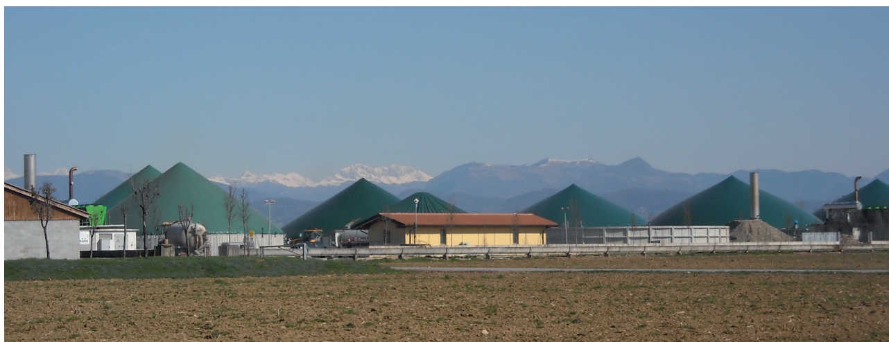
Figure 2.3.3. View of a collective treatment plant in Bergamo province (Martinengo, Lombardy, Italy).
