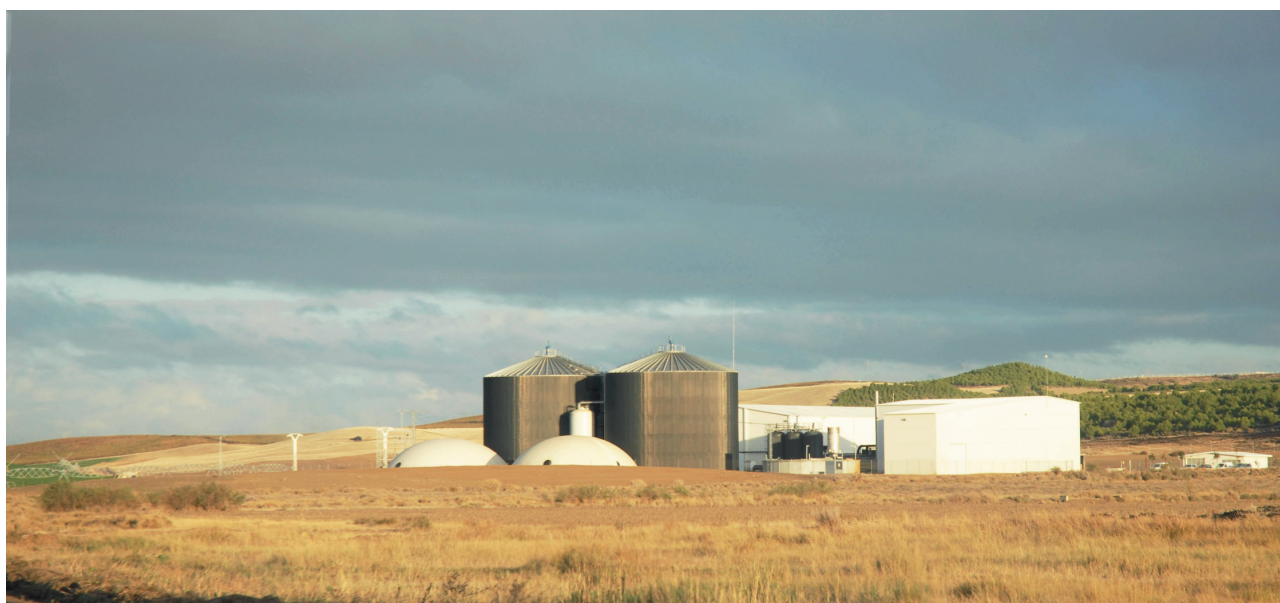
Figure 6.1.1. General view of the anaerobic digestion treatment plant in Caparroso (Navarra, Spain).
