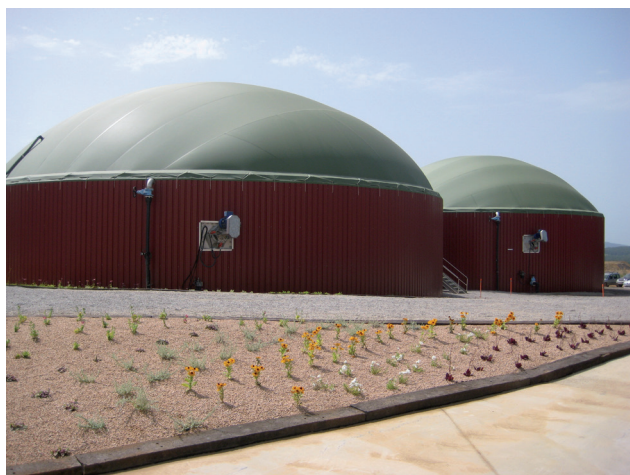
Figure 5.3.3. Anaerobic digestion plant at dairy cow farm (Catalonia, Spain)
