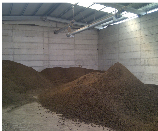
Figure 5.7.3. (Left) Dried digestate end-product. Green Energy farm - Brescia, Italy (CRPA, 2015).
