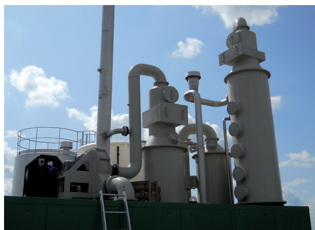
Figure 5.8.2. Ammonia stripping plant located in an agricultural biogas plant in Brescia, Italy - CRPA, 2015
