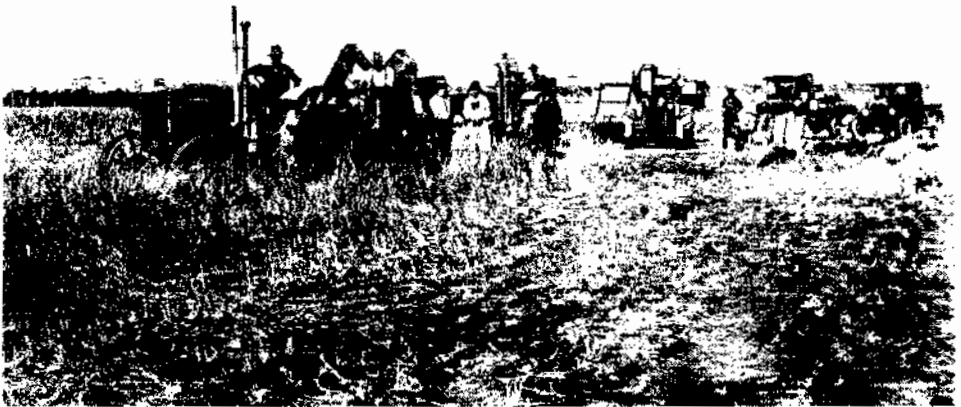
Plate 6: McMahon's machinery at work, 1927. (P. T. McMahon Collection: Courtesy Patricia Lawton)
