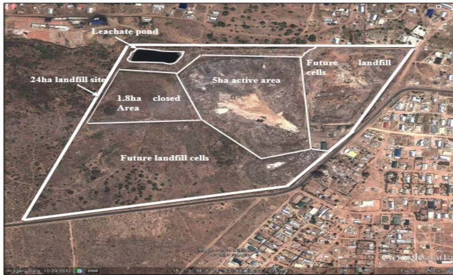
Figure 4.7: Aerial View of Landfill C
