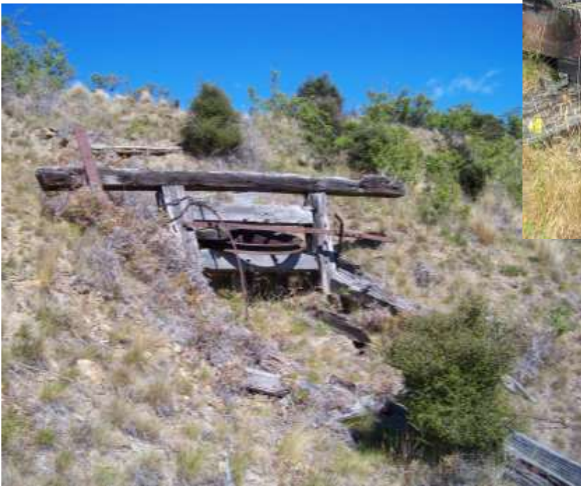
FIGURE 5 a & b Alta Aerial ropeway bucket and ropeway tension unit (1913), L.Carpenter 2011
