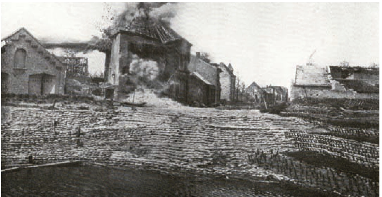
■ An emergency dam on the Nieuwpoort-Dunkirk canal at the moment of a bomb explosion (Kristof Jacobs, Nieuwpoort Sector 1917)
