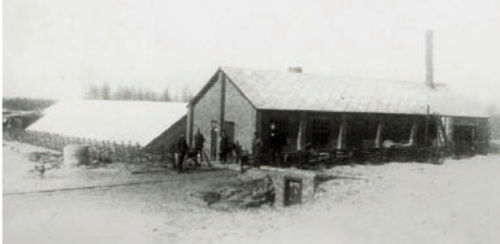
■ The pumping station for water collection in the Cabour dunes in the winter of 1917-1918 (Archives of Walter Lelièvre, Ramskapelle)
