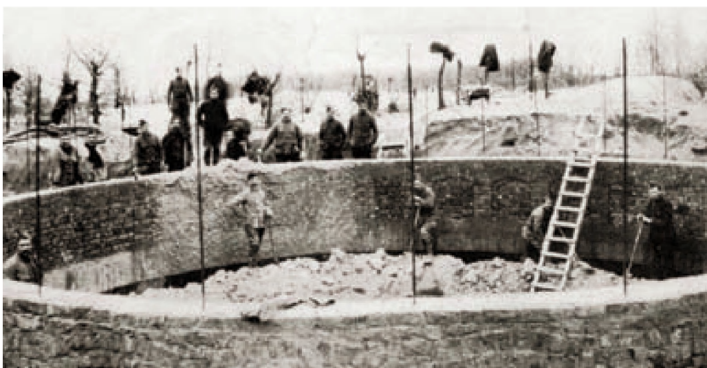
■ The construction of a water catchment hole in the winter of 1917-1918 (Archives of Walter Lelièvre, Ramskapelle)
