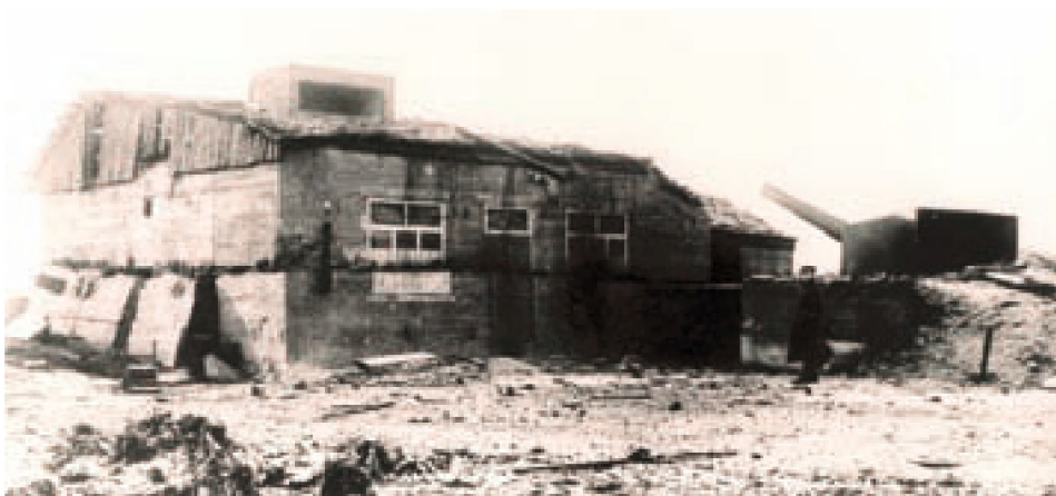
■ The Oldenburg Battery can confidently be considered an example of good camouflage. This is one of its bunkers, camouflaged as a farmhouse. Windows and doors were painted onto the concrete and a pitched roof was constructed on top. Note one of the artillery pieces on the right-hand side of the picture (CDH Evere, Foto Massot)
