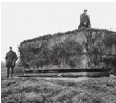
■ The observation and command bunker of the Aachen Battery was camouflaged with branches on top of the embrasure, since the bunker was one of the most conspicuous constructions of the complex when seen from the sea. The concrete reinforcement was added on top of the embrasure after the structure had been brought into use for the Deutschland Battery at Bredene in order to better protect the expensive equipment. This picture was taken after the war during a visit by American soldiers (Imperial War Museums, MH 30839)
