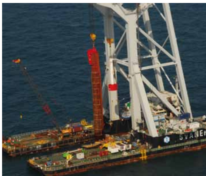
Jacket pin pile (left) and monopile (right) driving preparation at the Thorntonbank and Bligh Bank.
