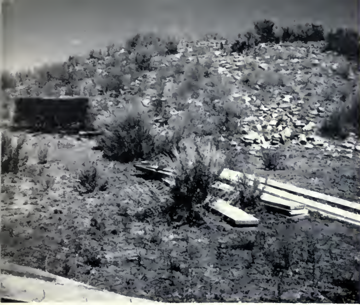
Left, Lowry Pueblo as it appeared forty years ago, when the author began to dig. Below, restored Lowry Pueblo, a National Historical Landmark. The two photographs were taken from nearly the same spot.
