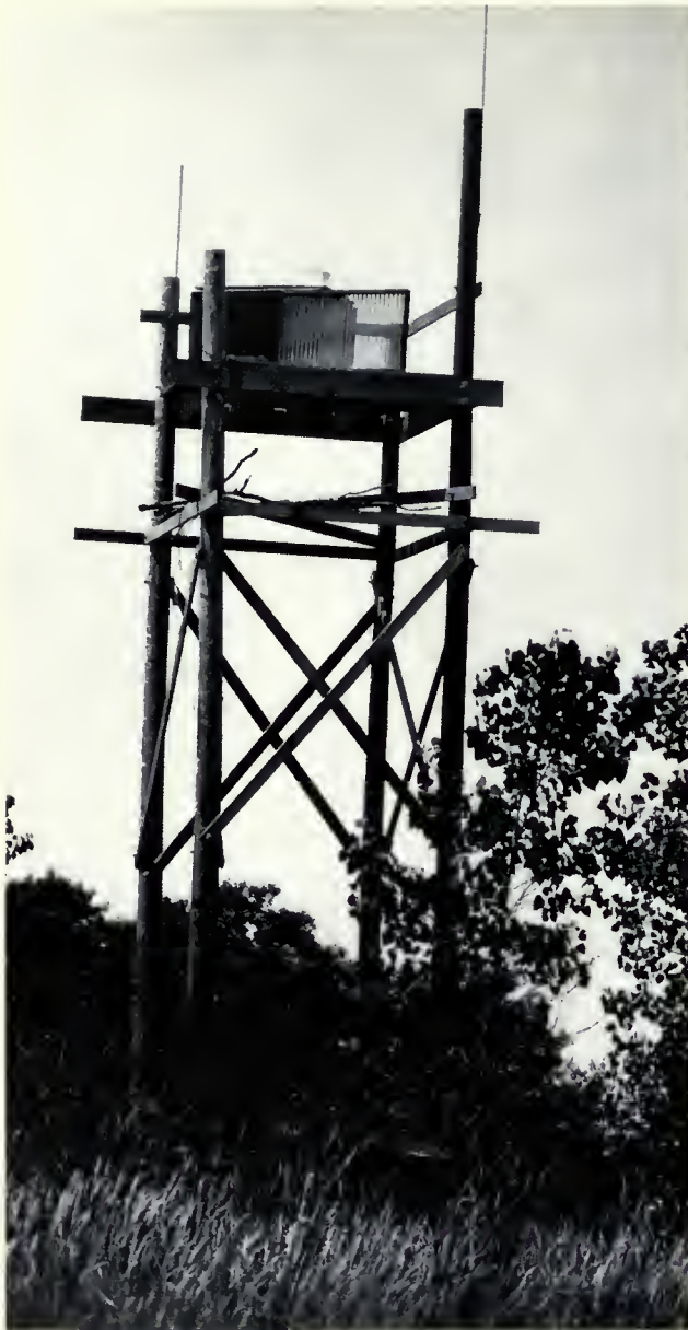
Peregrine release tower at Illinois Beach State Park. Shields near the bottom of the support posts prevent raccoons from climbing the tower. Tower was built courtesy of the Telephone Pioneers of America.
