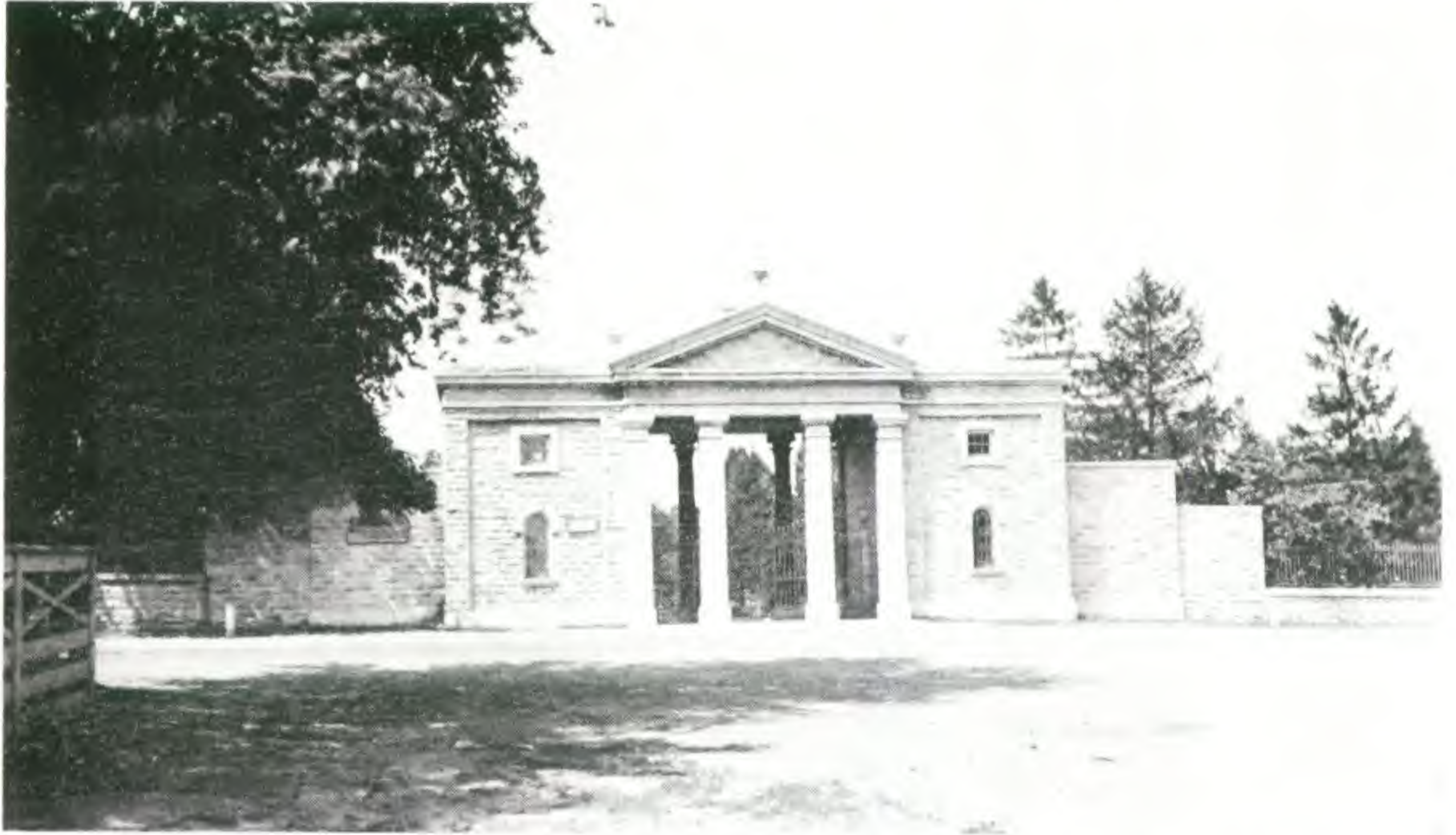
Mr. Shaw's main gate as it looked during his last years. His original stones above the entrance, proclaiming that this is the MISSOURI BOTANICAL GARDEN, were incorporated in the present entrance, completed shortly before World War I.
