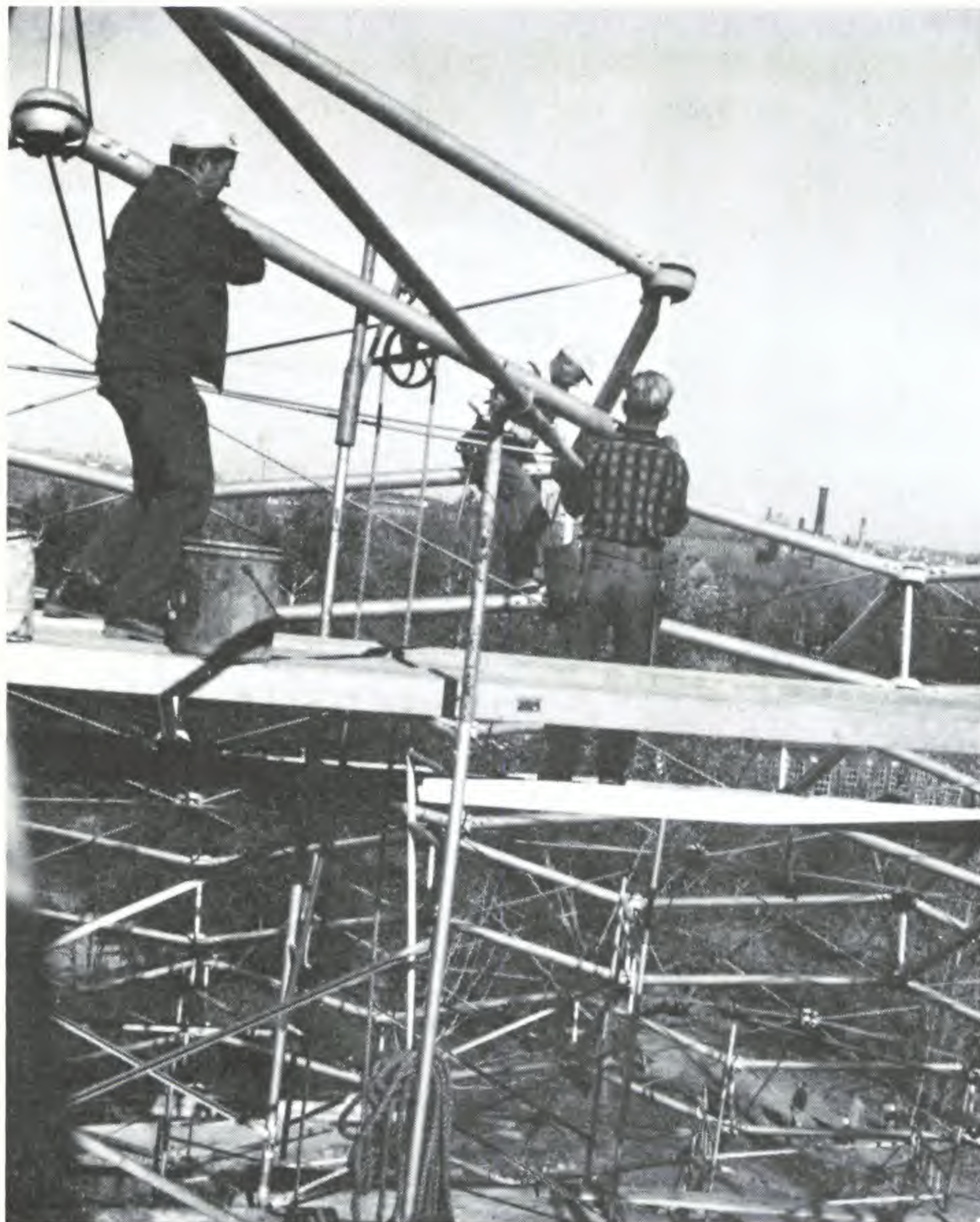
Assembling the dome. Note how comparatively light are the big tubes of aluminum alloy.
