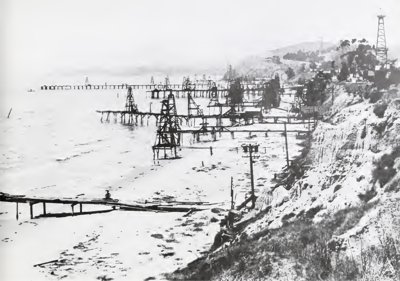
Among the first wells drilled over water are these in the Summerland field, California. Just south of Santa Barbara, this 100-acre field produced from a depth of 210 feet. The photo was taken circa 1920. (Courtesy of World Oil)
