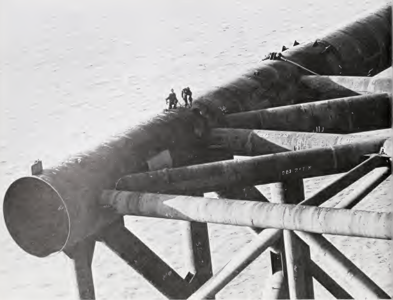
A 4,000-ton drilling platform is readied for sinking to the bottom of the middle ground shoals of Cook Inlet, Alaska. (Photo by Joe Rychetnik/PR)
