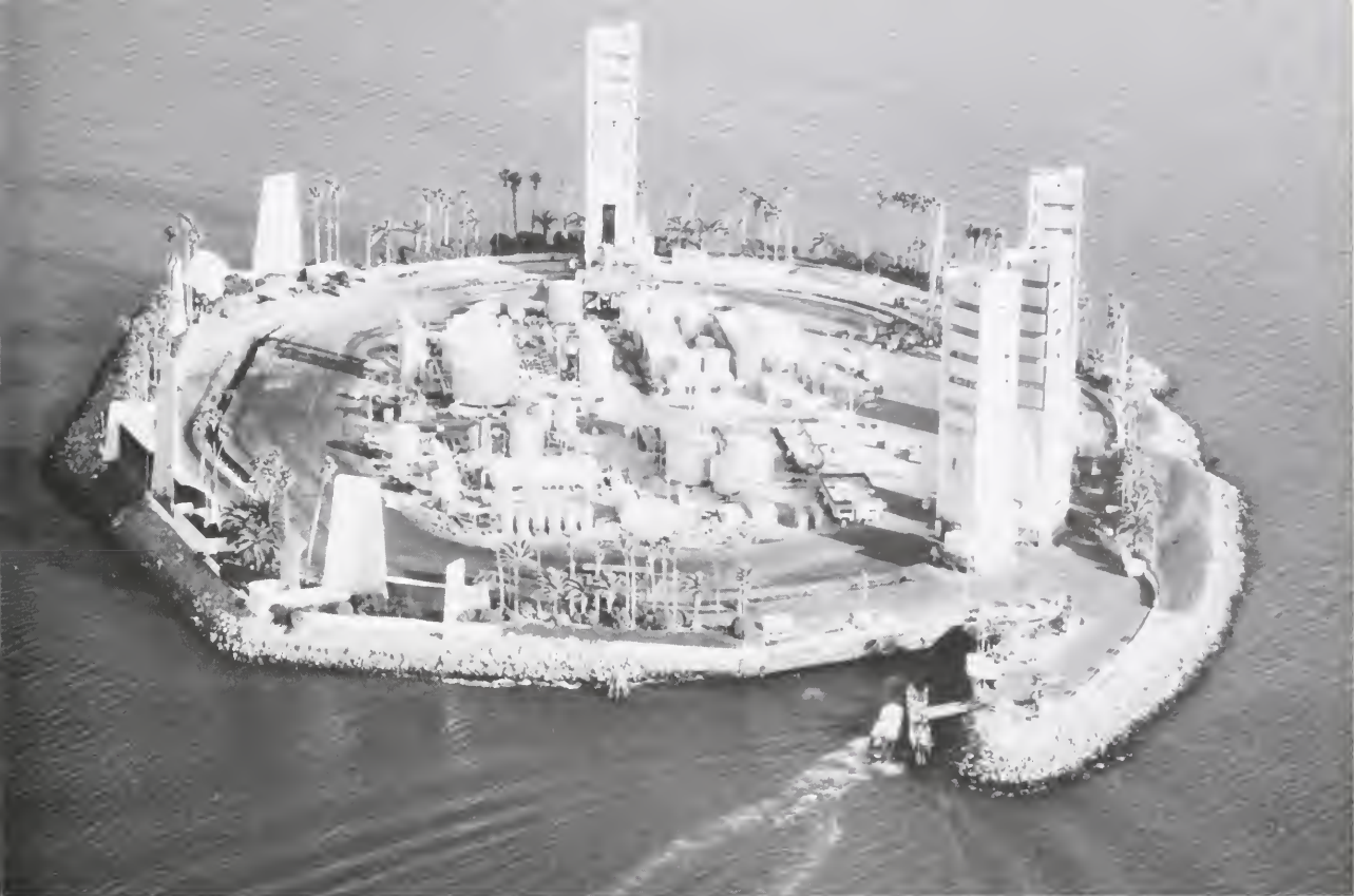
"Beautified" artificial island for oil and gas operations located in Long Beach Harbor, California. (Photo by Steve Proehl/PR)
